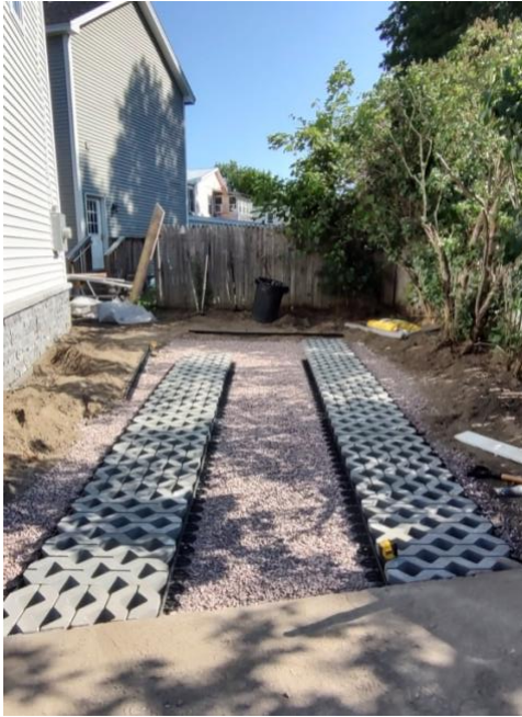
[left] Permeable ribbon strip driveway installation. [Right] Driveway infiltration trench.
