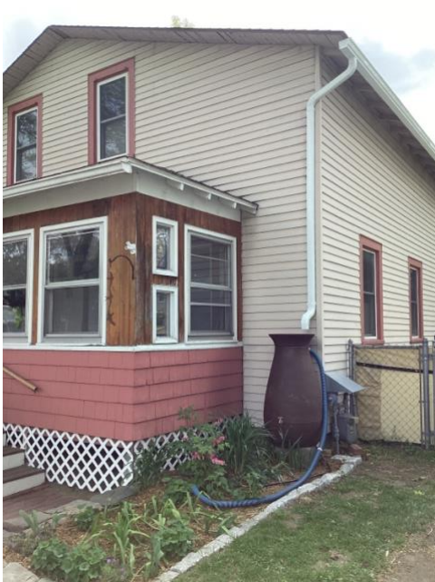
[left] Gutter and rain barrel. [right] Rooftop disconnection.
