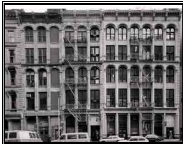
Figure 115: Historic TriBeCa block in New York City that maintains its fire escapes (Allen, Oliver E., “Architecture,” Tribeca Organization, http://www.tribeca.org/history/architecture.aspx )
