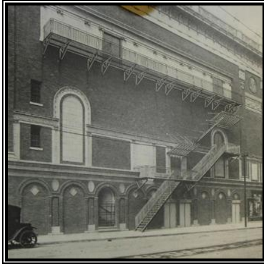
Figure 97: J.E. Bolles, No. C 3760 Theatre Fire Escape (J.E. Bolles Iron and Wire Works. Sectional Catalogue . Detroit: The Firm, 1913: 5)
