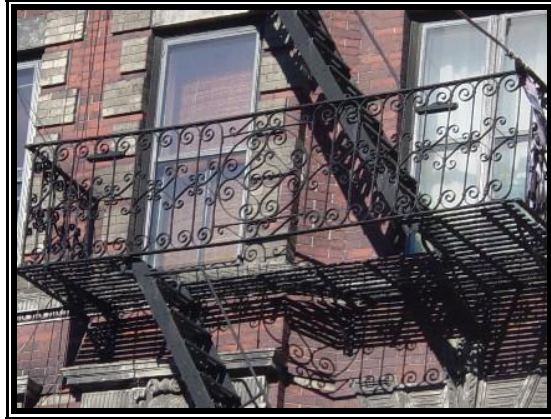
Figure 118: Ornamental fire escape at 169 Sullivan Street, South Village, New York City (Greenwich Village Society for Historic Preservation, “South Village - A Distinguished History Largely Unrecognized,” New York City, http://www.gvshp.org/south_village948.htm )
