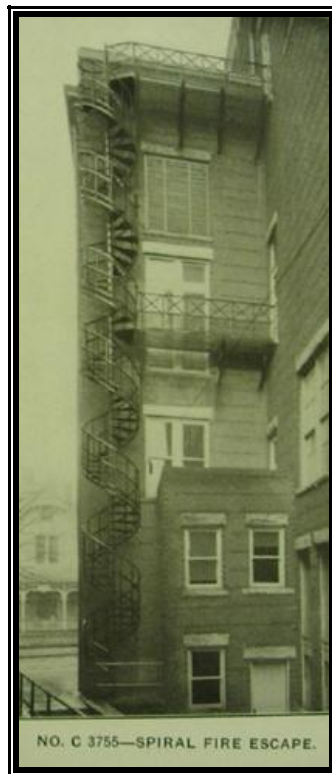
Figure 96: J.E. Bolles, No. C Spiral Fire Escape (J.E. Bolles Iron and Wire Works. Sectional Catalogue . Detroit: The Firm, 1913: 4)
