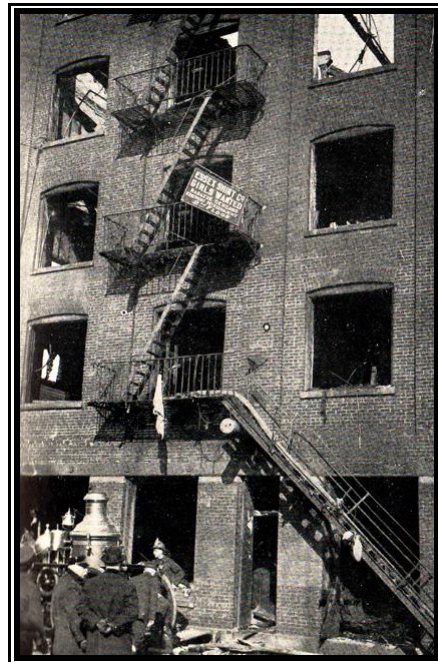
Figure 22: Flames shot out the window at this deadly factory fire, rendering the fire escape impassible. (“Two Factory Fire Holocausts,” Quarterly of the National Fire Protection Association 9 (1916), 273.)
