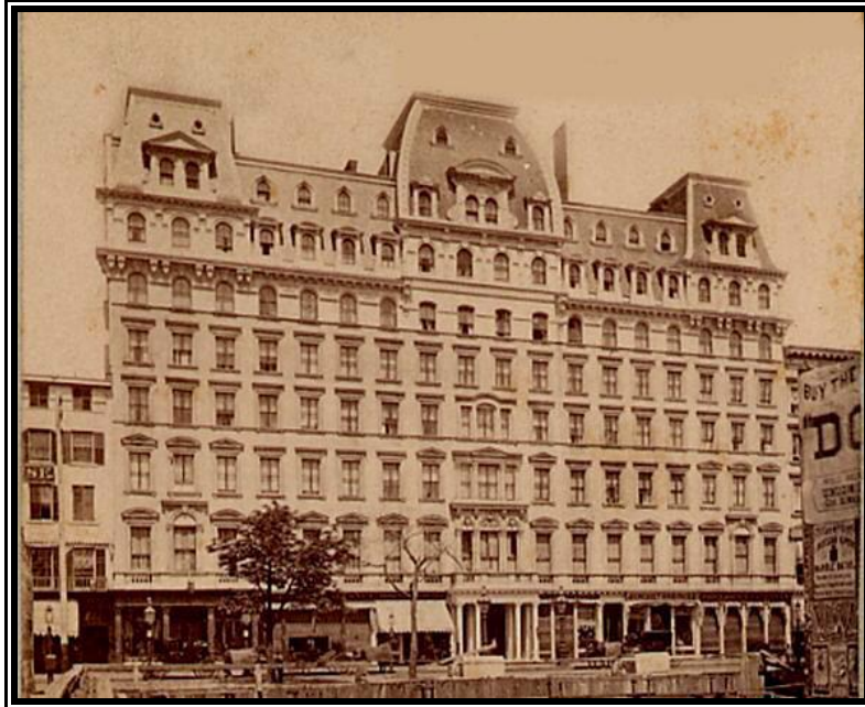
Figure 15: Broadway Central Hotel prior to the erection of fire escapes. (Courtesy of “Randall’s Lost New York City,” http://www.lostnewyorkcity.com , accessed October 21, 2005)
