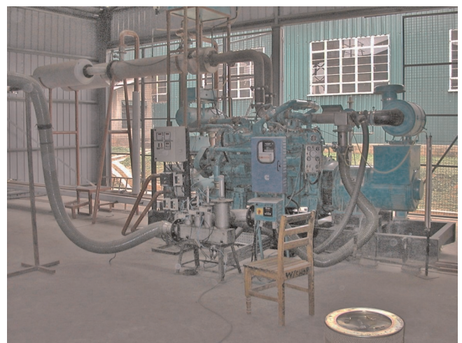
Figure 4. 250 kW producer-gas engine with heat exchangers (upper left corner at exhaust pipe, heat exchanger at cooling cycle covered by control units) at Muzizi Tea Estate
