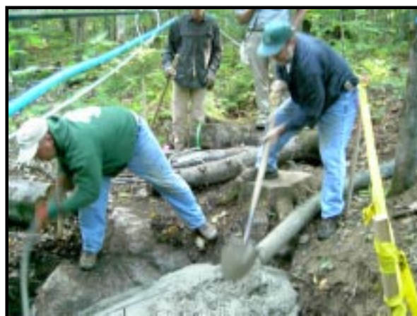
Marc Eisenhower and Carl Waite spreading concrete in the anchor holes.
