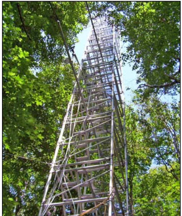
VMC’s 66-foot walk-up forest canopy tower at Proctor Maple Research Center in Underhill, Vermont.
