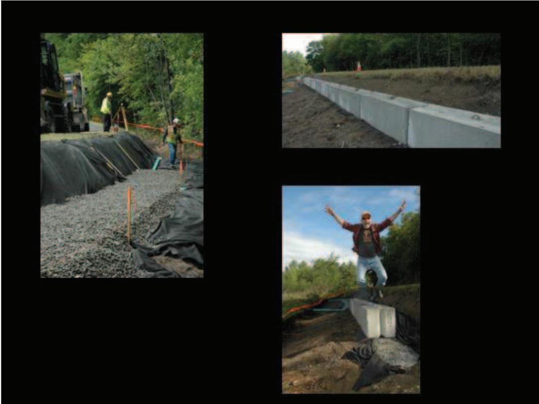
Figure 7. Construction of the Monkton amphibian underpass
