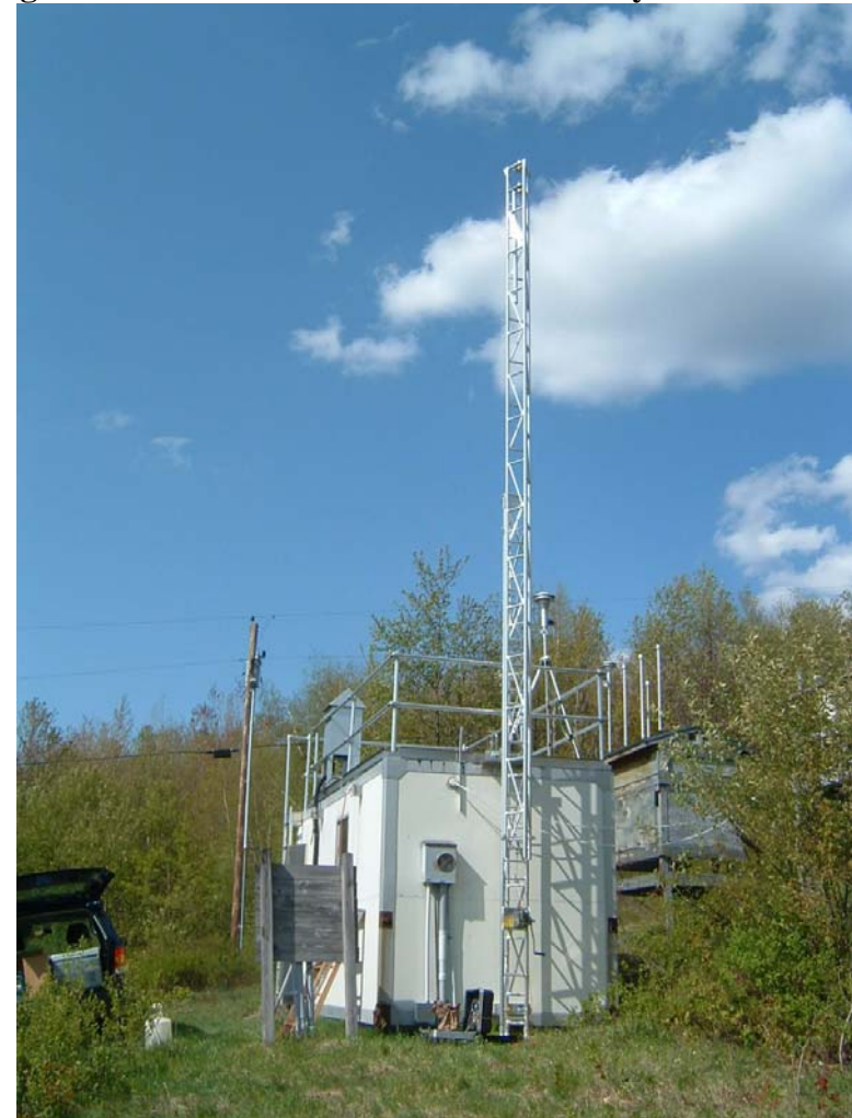
Figure 7 - Underhill Installed 10 Meter NOy Tower
