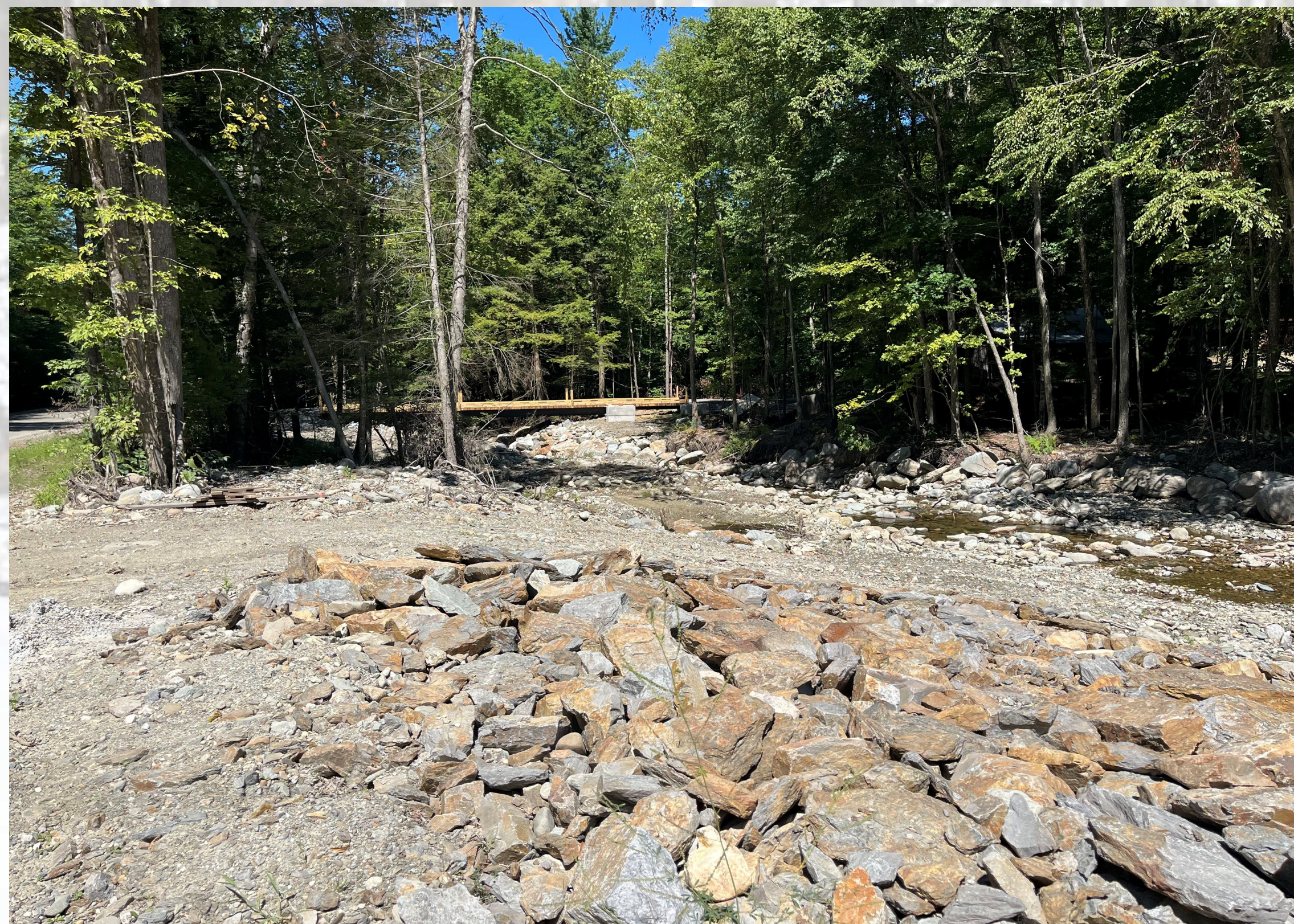
Extensive flood damage along lower Ireland Road in Starksboro. Reducing the volume and velocity of storm flow starts in headwater forests. Most soil erosion and stormwater runoff from forests comes from access roads.
