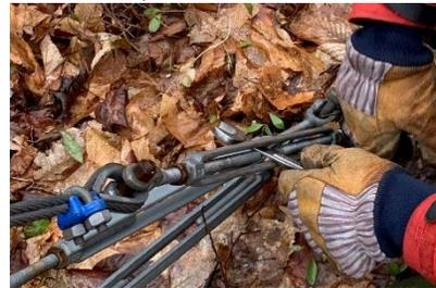
Figure 2. Tensioning the wire by rotating the turnbuckle, using the wrench for leverage.
