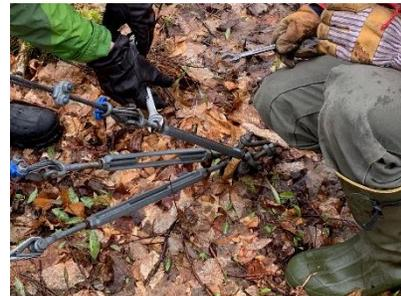
Figure 1. Loosening the lock-nuts above and below the turnbuckle.
