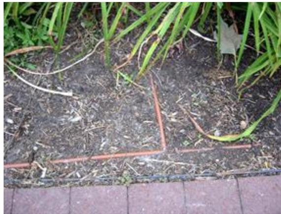
**Figure 9 – Drip Irrigation**
