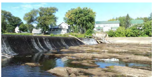
The Swanton Village Dam in 2015
