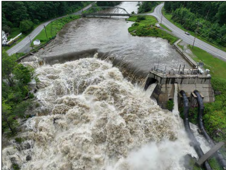
Figure 4-9 Fairfax Falls hydroelectric dam overtopping from July 2023 flooding
