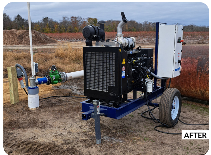
(Before) The farm’s five pumps were bringing in enough water, but the farm manager knew there was a way to reduce fuel use and improve efficiency. (After) New electric pumps, powered by new Tier 4 diesel generators are saving the farm money and reducing their emissions. Photos by Michelle Pedano, USDA-NRCS
