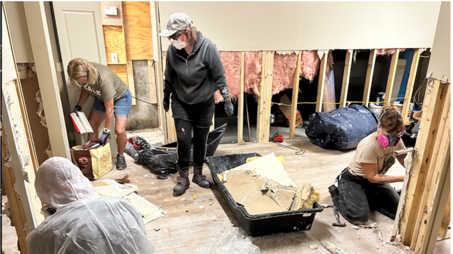
Community members remove drywall from a home damaged in the July 2023 floods. NEKO assembled mutual aid crews to clean and gut flooded homes across the region in both 2023 and 2024. Photo Credit: NEKO.
