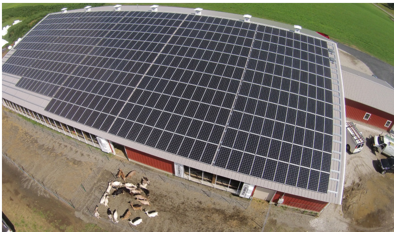
A 150kW system with 572 solar panels, utilizing a south facing roof on the Ayers Brook Goat Dairy in Randolph, VT. Photo Source: Aegis Renewable Energy
