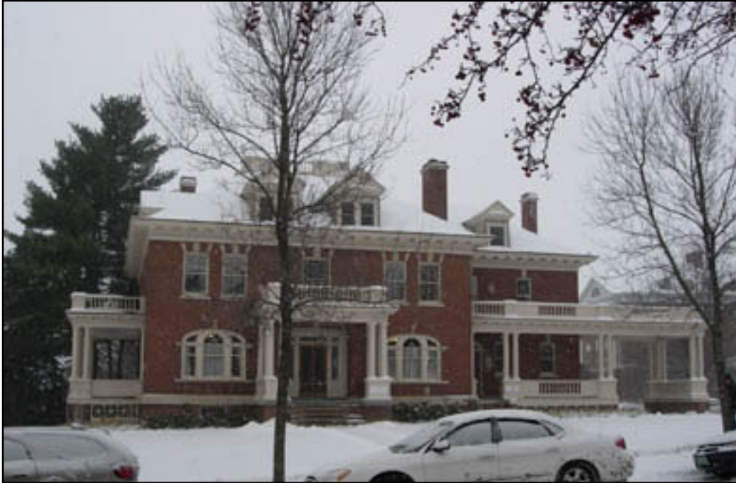
Figure 4.15: This photograph, taken in early December 2007, shows the University of Vermont's E.J. Booth House after green rehabilitation. Work to reopen the side porch (left) and to recreate the porte-cochere (right) were part of plans to restore the building's primary façade to its 1950 appearance. View looking northeast. Author photograph.
