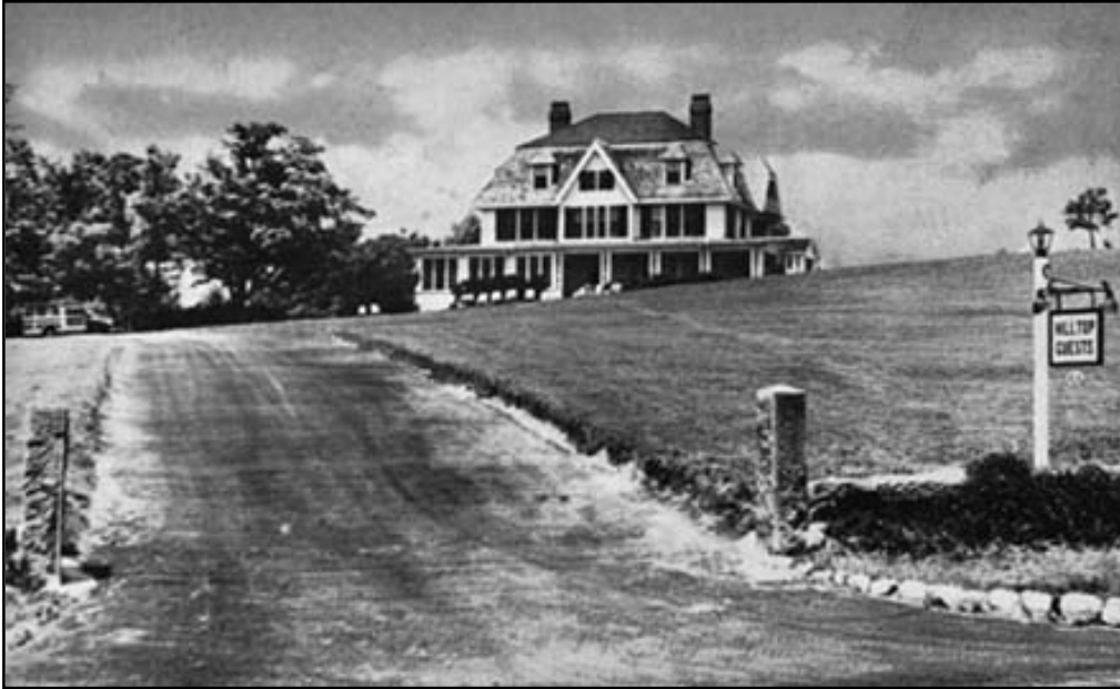
Figure 2.15: Photograph showing Hilltop House, a hotel that occupied the historic Helen Turner House in Falmouth, Massachusetts, from the 1950s through the 1980s. View looking north. Circa 1965. Courtesy of Arcadia Publishing. Reprinted with permission from Images of America: Falmouth , by Ann Sears and Nancy Kougeas. Available from the publisher online at www.arcadiapublishing.com or by calling 888-313-2665.
