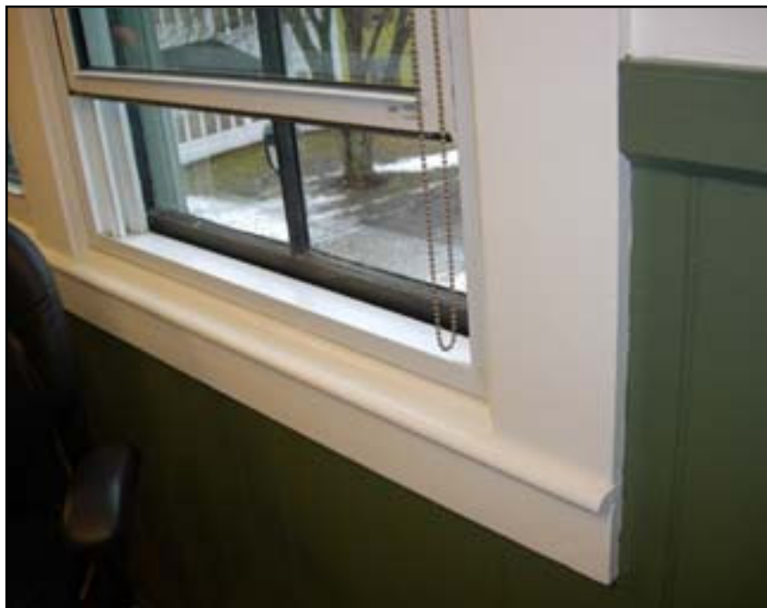
Figure 4.12: “Super-insulating” windows were installed behind historic windows during Debevoise Hall’s green rehabilitation. Winter 2006. Author photograph.
