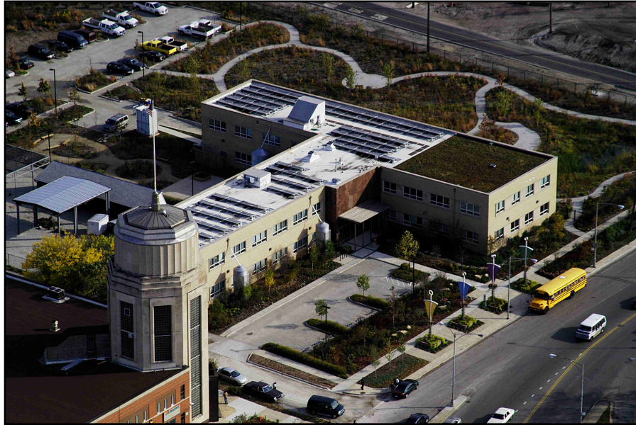
Figure 3.3: Aerial photograph of the rehabilitated Chicago Center for Green Technology. Note the building's roof-mounted photovoltaic (PV) panels and vegetated roof. View looking southeast. Circa 2002. Courtesy of Chicago Department of Environment. Used with permission.
