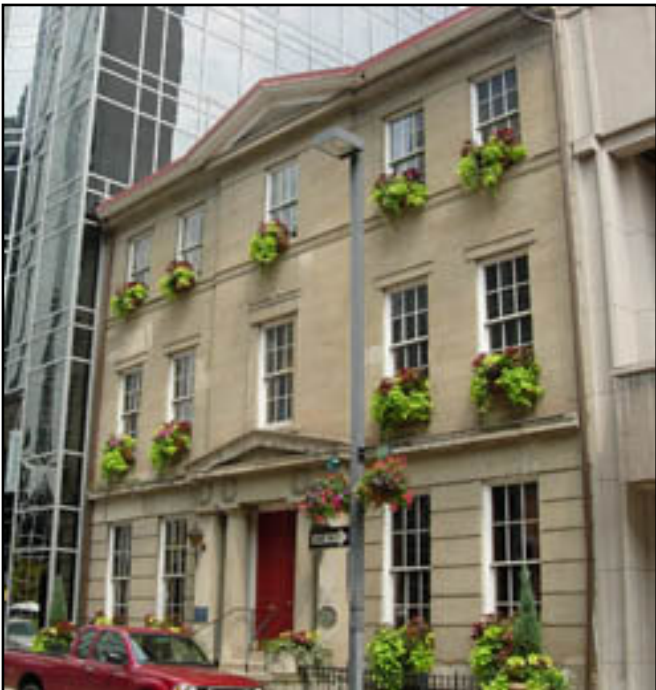
Figure 2.6: Burke Building, headquarters of the Western Pennsylvania Conservancy, in downtown Pittsburgh, Pa. View looking northeast. Summer 2005. Author photograph.
