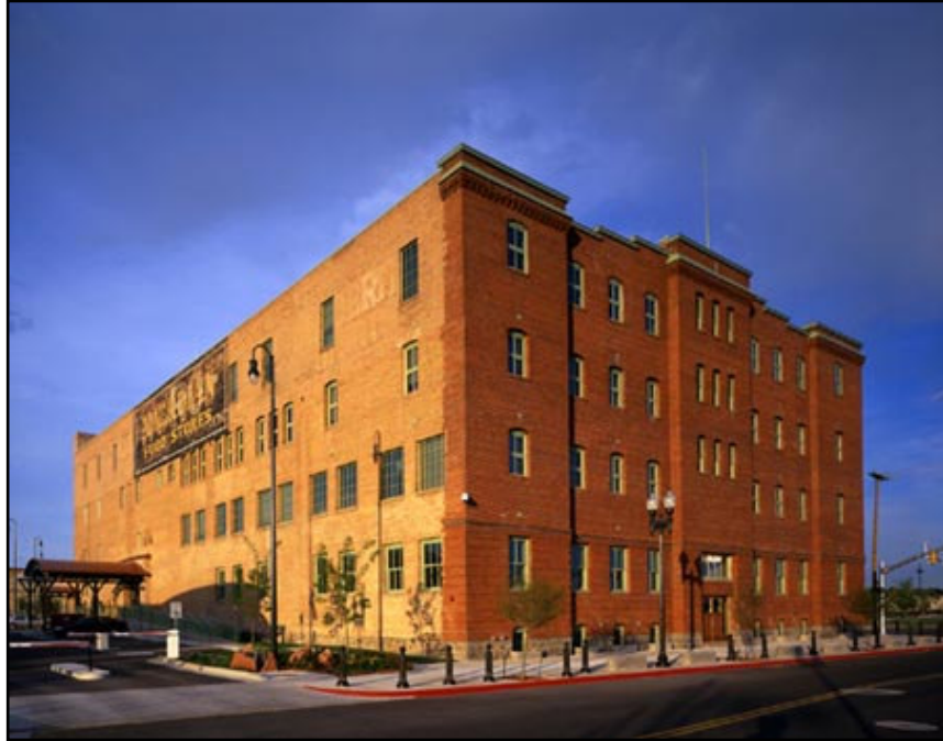
Figure 4.19: Ogden, Utah’s historic Scowroft Warehouse (1906) underwent a LEED-NC 2.0 “Silver” rated rehabilitation, reopening in 2004 as office space for the U.S. Internal Revenue Service. View looking southwest. Circa 2004. Photograph © Paul Richer. Courtesy of Cooper Roberts Simonsen & Associates Architecture. Used with permission.
