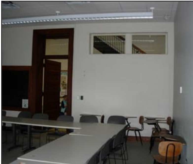
Figure 2.14: Typical post-rehabilitation classroom in Barney-Davis Hall, with historic chalkboard, door with transom, and woodwork as well as new transoms, lighting fixtures, ceiling, and furniture. Fall 2006. Author photograph.
