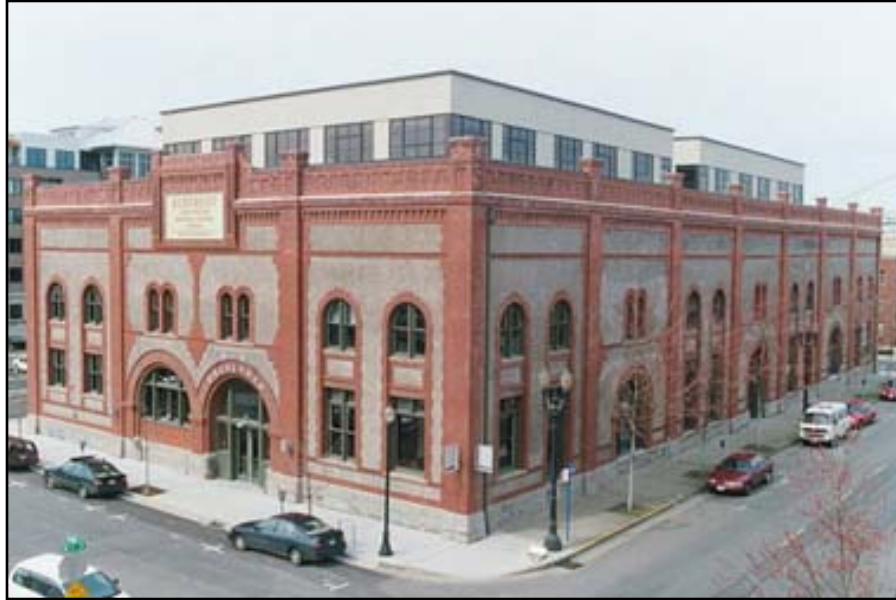
Figure 3.5: Opened in 2001, the Jean Vollum Natural Capital Center houses office and retail space for private, nonprofit, and government tenants. Note the new rooftop penthouse's prominence, which the National Park Service ruled violated the Secretary's Standards for Rehabilitation . View looking northwest. Circa 2001. Courtesy of Interface Engineering. Used with permission.
