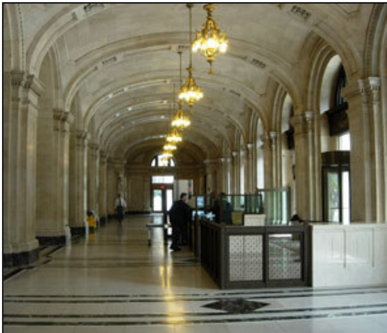
Figure 4.22: View of the Metzenbaum U.S. Courthouse’s historically significant public entry lobby after the 2004-2005 rehabilitation. Summer 2005. Author photograph.
