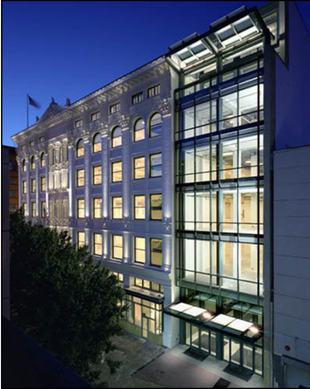
Figure 4.1: In 2002, the Harry and Jeanette Weinberg Foundation rehabilitated the circa 1889 Stewart's Department Store Building as LEED-NC 2.0 "Certified" office space. Circa 2002. Image Courtesy of Design Collective, Inc. / Bob Creamer Photography. Used with permission.
