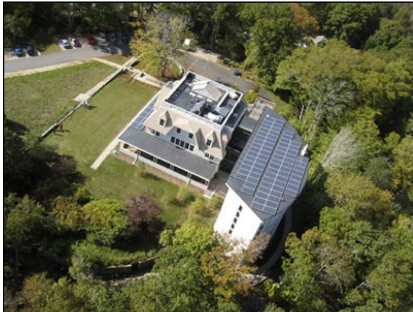
Figure 2.20: Aerial photograph of Woods Hole Research Center's Gilman Ordway Campus, showing the renovated Helen Turner House (center) and new addition (right). View looking southwest. Fall 2004. Photograph by Charles Benton. Used with permission.
