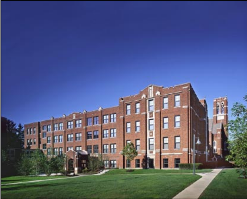
Figure 4.3: Post-rehabilitation view of the historic Felician Sisters motherhouse in Coraopolis, Pennsylvania. The building is LEED-NC 2.0 “Gold” rated. Circa 2003. Courtesy of Perkins Eastman Architects. Used with permission.
