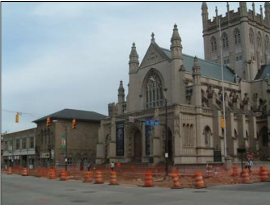
Figure 4.2: A green rear addition (not shown here) links the Gothic Revival style Trinity Episcopal Cathedral (right) with several historic commercial storefronts (left) to form the Trinity Commons complex in downtown Cleveland, Ohio. View looking southeast. Spring 2007. Author photograph.
