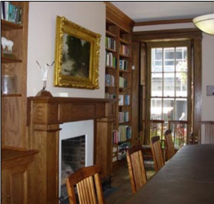
Figure 2.8: The Burke Building's library features historic interior window shutters and built-in bookcases made from historic oak salvaged during the rehabilitation. Summer 2005. Author photograph.
