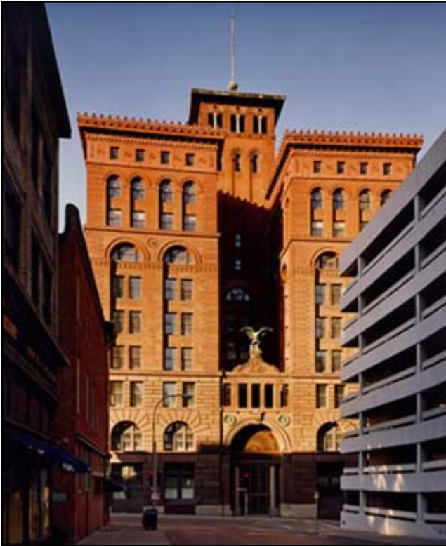
Figure 2.1: The historic New York Life Building, in downtown Kansas City, Missouri, was rehabilitated in 1997. Sustainable features include daylighting strategies, energy conservation measures, and low VOC construction materials. View looking north. Circa 1997. Photograph by Mike Sinclair. Courtesy of Gastinger Walker Harden Architects. Used with permission.
