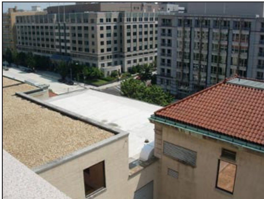
Figure 3.22: A reflective roof of light-colored pebbles and a white membrane on the "M" Street and 1933 buildings helps reduce the National Geographic Society's contribution to Washington's urban heat island effect. The reflective roof surfaces are not visible from street level. View looking northeast. Summer 2005. Author photograph.
