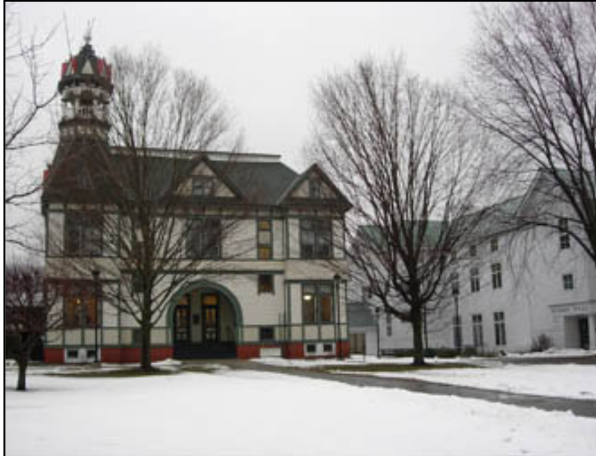
Figure 4.11: Vermont Law School’s rehabilitated Debevoise Hall combines energy efficiency, water reduction, and other sustainable features with sensitive historic preservation. View looking northwest. Winter 2006. Author photograph.
