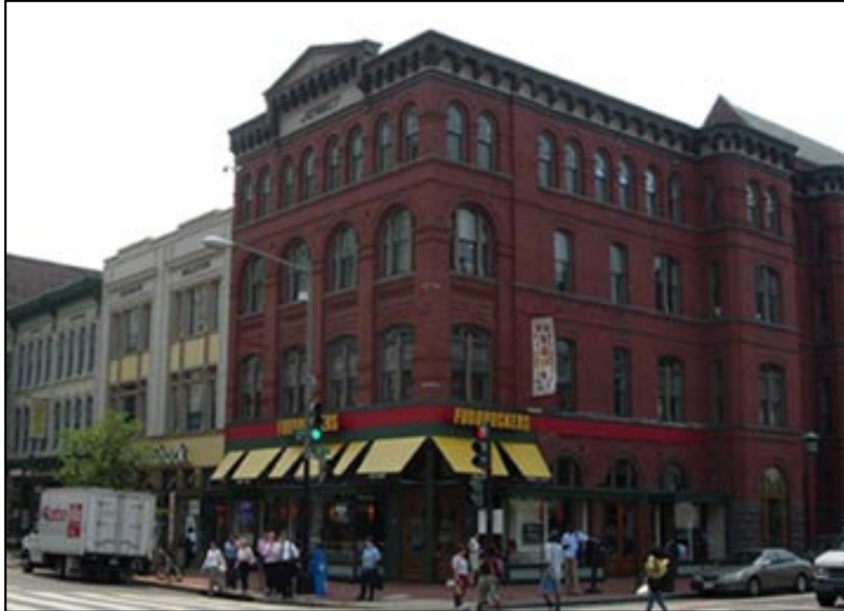
Figure 2.3: Greenpeace-USA headquarters (second floors in connected buildings), summer 2005, in Chinatown, Washington, D.C. View looking southwest. Author photograph.
