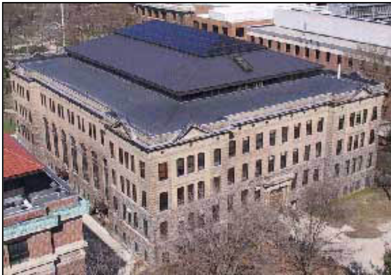
Figure 3.8: Aerial photograph of Samuel T. Dana Building after the central atrium has been enclosed. View looking southwest. April 2001. Courtesy of School of Natural Resources, University of Michigan. Used with permission.
