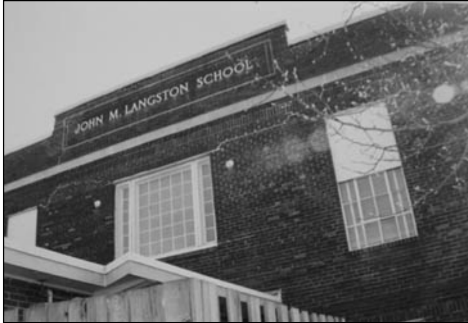
Figure 3.1: Pre-demolition documentation photograph of the John M. Langston School's historic front parapet. View looking east. Circa 2002. Photograph by Steve Stricker. Source: Arlington County Historic Preservation Commission. (Photographs submitted by Arlington County Public School System to Arlington County Historic Preservation Commission on February 5, 2002, under Special Use Permit #U-3007-01-1.)
