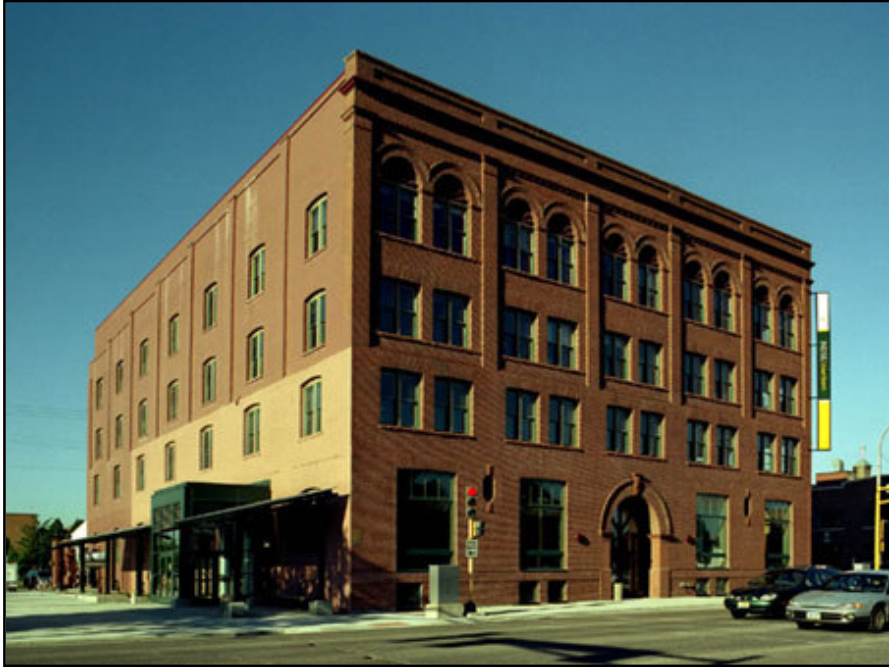
Figure 4.13: Photograph of North Dakota State University's Downtown Campus. The building's rehabilitation earned federal historic preservation tax credits (RITC) and a LEED-NC 2.0 "Certified" rating. View looking south. Circa 2004. Photograph by Saari and Forrai Photography. Courtesy of Michael J. Burns Architects, Ltd. Used with permission.
