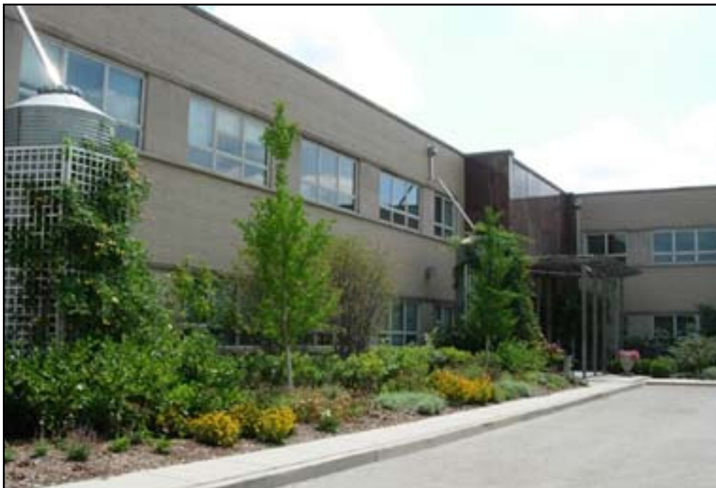
Figure 3.4: Front façade of the Chicago Center for Green Technology. Note the rain water cistern (left), partially screened by flowering vine vegetation growing on latticework. View looking south. Summer 2005. Author photograph.
