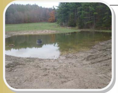
Rehabilitated farm pond with overflow and water intake structure installed. Fence was built to exclude livestock from pond and stream.
