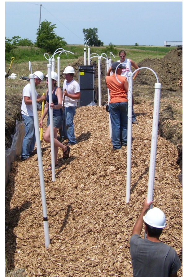
Installing monitoring wells in a bioreactor in Illinois.
