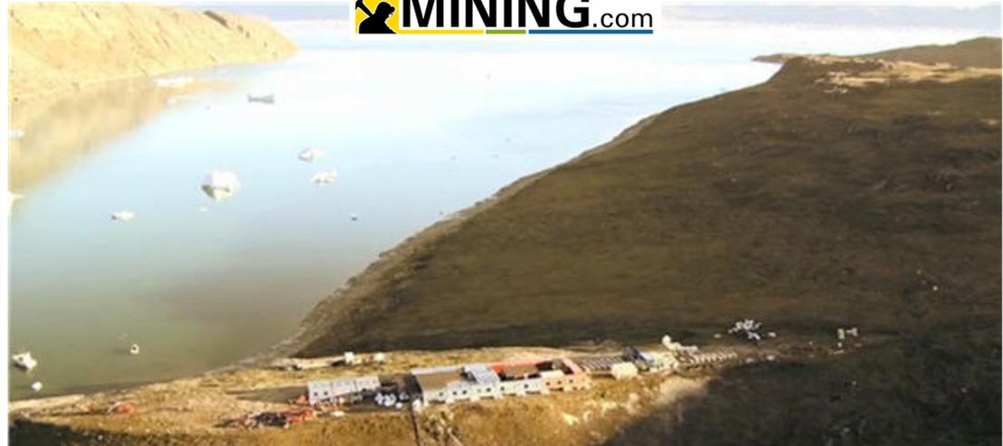
The Isua project will comprises of a mine, processing plant and 105km concentrate pipeline which connects the plant to a deepwater port capable of year round loading of 250,000t ships. Image from [London Mining corporate video](#).
