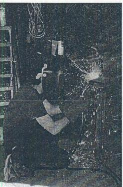
Many farm workers do their own welding to assist with machinery repair. Welding consists of holding the welding rod against the item to be repaired and could involve some prolonged positioning such as bending. A welding rod is of minimal weight but the item being welded may be heavy. Items to be welded can occasionally be pushed or pulled in order to position for welding and the weight can vary.
