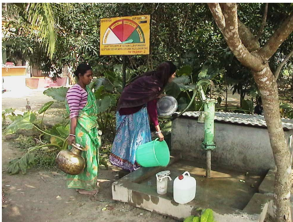
Fig. 1. Newly installed shallow dugwell with hand pump extraction of water to replace tubewell with water arsenic concentration of 220 \mu\text{g/l} . Arsenic concentration in this dugwell was 6 \mu\text{g/l} , but concentrations in such dugwells may be in range from 2 to 50 \mu\text{g/l} .
