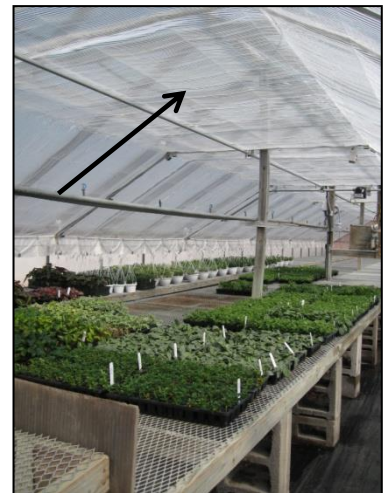
Fig. 13. Thermal curtain used for shade to cool plants on a hot sunny day.
