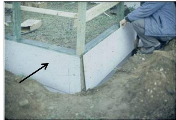
Fig. 8. Insulate the perimeter foundation with foam board.
