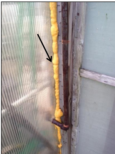
Fig. 2. Corner joint weather-proofed with expandable foam spray insulation.
