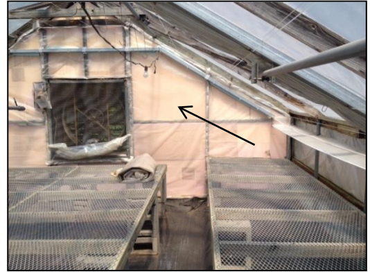
Fig. 4. End wall insulated and covered with a layer of poly.
