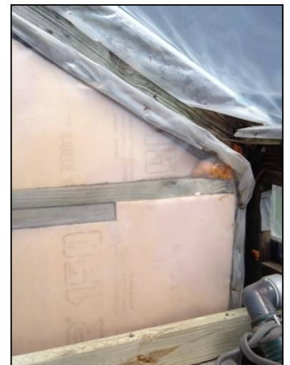
Fig. 10. Insulated and poly-covered end wall.
