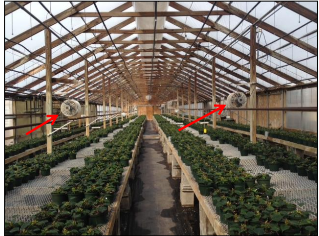
Fig. 12. Properly installed horizontal air flow fans (red arrows). There should be one or more on each side arranged to keep air moving in a circular manner.
