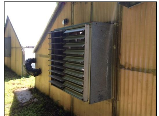
Fig. 6. Fans of this type should be sealed from the inside with foam board or poly.
