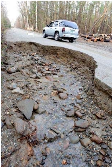
Figure 6 Road washouts due to flash flooding between Jericho and Underhill, VT [Photo credit: The Burlington Free Press]
