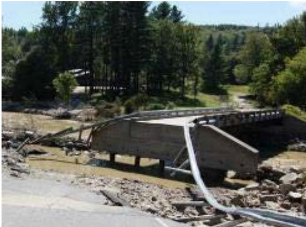
*(a) Scour behind an abutment of a bridge in Ludlow, VT (source: Burlington Free Press)*
