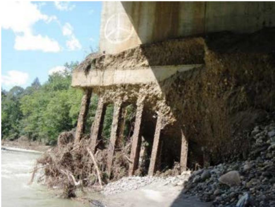
*(b) Dummerston VT30-B9 Bridge: scour beneath the concrete spread footing, with settlement resulting in the cracking of the foundation.*
