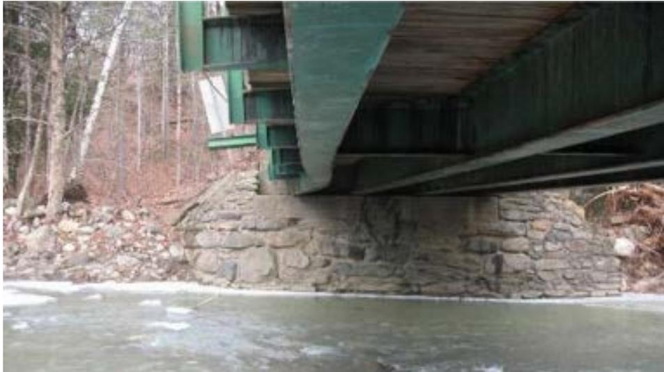
*(b) Marlboro C3014-B23 Bridge: damage to the main beam of the bridge from debris impact*
