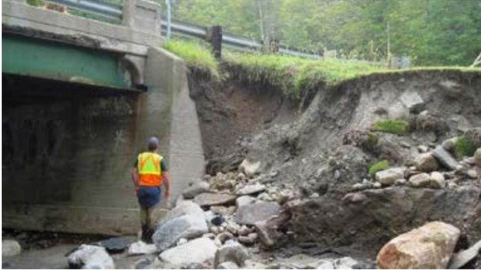
*(a) Wardsboro VT100-B68 Bridge: flanking erosion behind the abutment, and minor scour to the footing*
