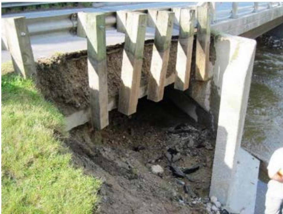
*(b) Jamaica VT30-B40 Bridge: flanking behind the abutment undermining the approach slab*
