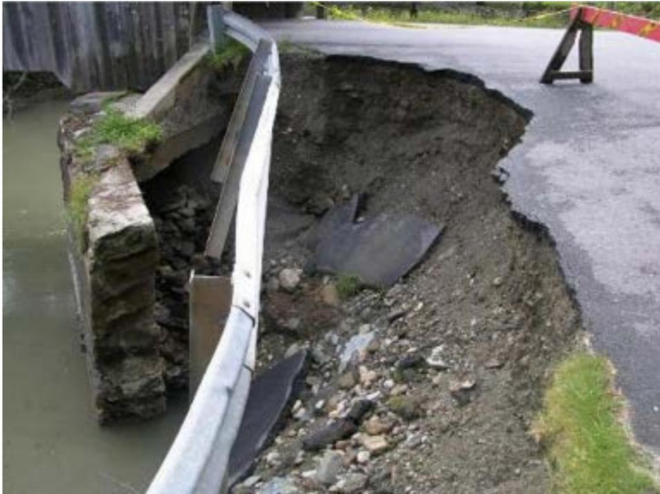
*(b) Warren FAS188-B6 Bridge: Channel erosion and flanking behind the wingwall, with scour hole at the toe*
