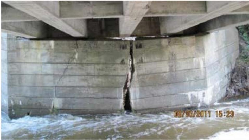
*(a) Brownington C2001-B9 Bridge: fracture to the foundation, due to scour beneath the footing and settlement of substructure*
