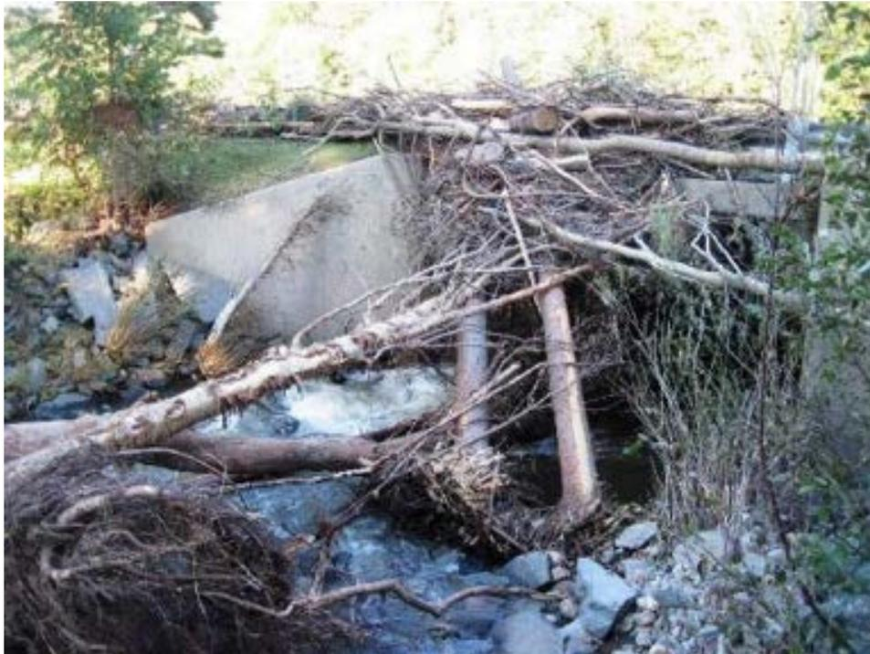
*(b) Wilmington VT100-B53 Bridge: obstructions at a small single span resulting in blockage and overtopping*
