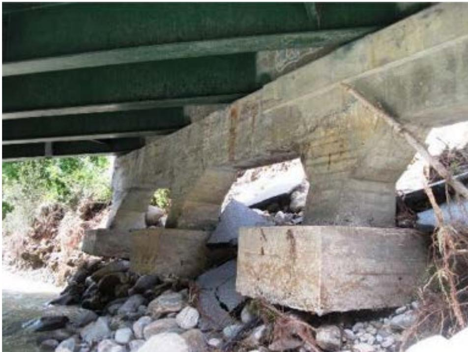
*(b) Jamaica VT30-B78 Bridge: flanking behind the wingwall abutment, with scour beneath the bridge foundation, with no apparent damage to the concrete foundation, and no major settlements to the foundation*
