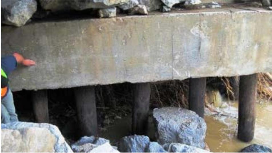
*(a) Clarendon US7-B96 Bridge: scour beneath the foundation, exposing several feet of wooden piles*
