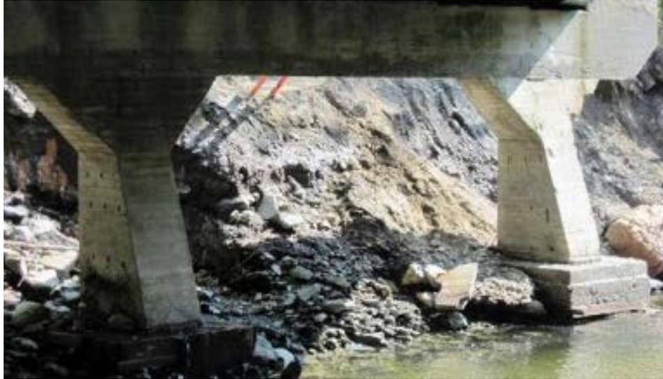
*(a) Halifax C2001-B17 Bridge: loss of original riprap and backfill, resulting in the free standing abutments and scour to beneath the footing of the spread footing base*
