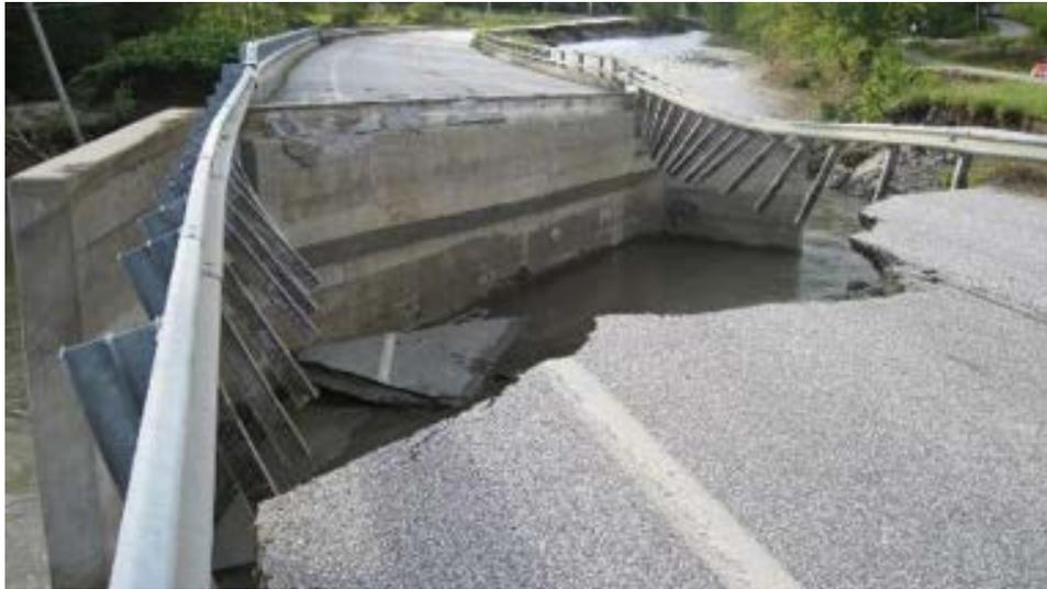
*(a) Braintree VT112A-B6 Bridge: erosion behind the wing-walled abutment, with complete loss of the bridge approach*
