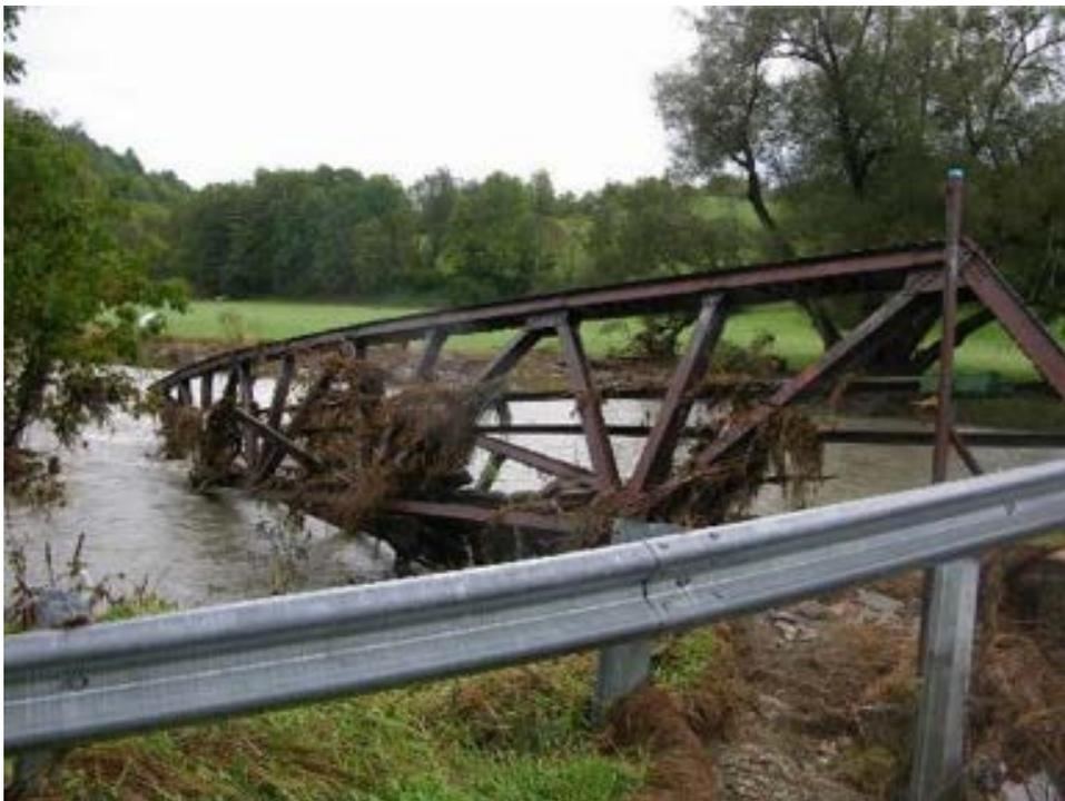
*(b) Moretown C3024-41 Bridge: collapse of the steel truss bridge from the apparent loss of one of the bridge foundations*
