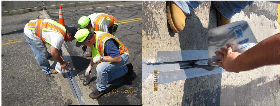
Figure 5. Sealing of the Bridge Joint in CT
