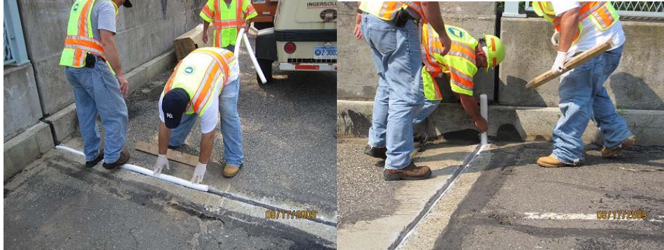
Figure 4. Placement of Backer Rod into Joint in CT
