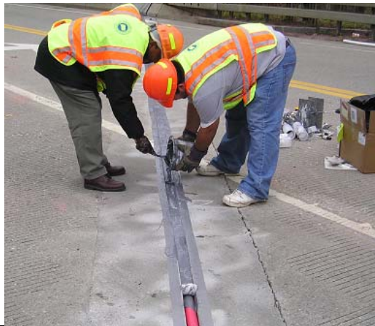
Figure 20. Sealing of New York Expansion Joint
