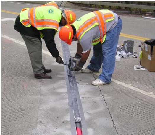
Figure 20. Sealing of New York Expansion Joint
