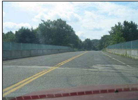
Figure 3. Candidate Bridge in Mansfield, Connecticut
