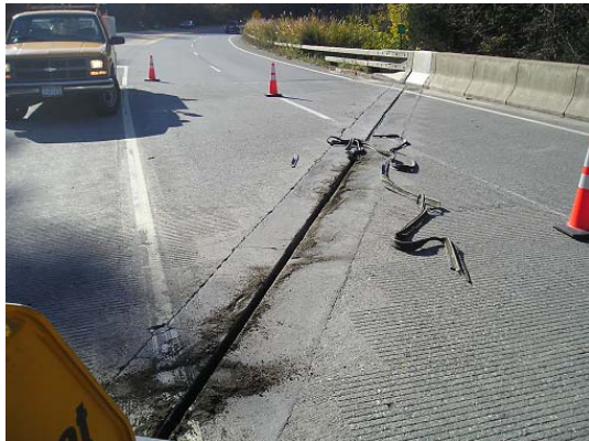
Figure 18. Candidate Bridge in Dover Plains, NY
