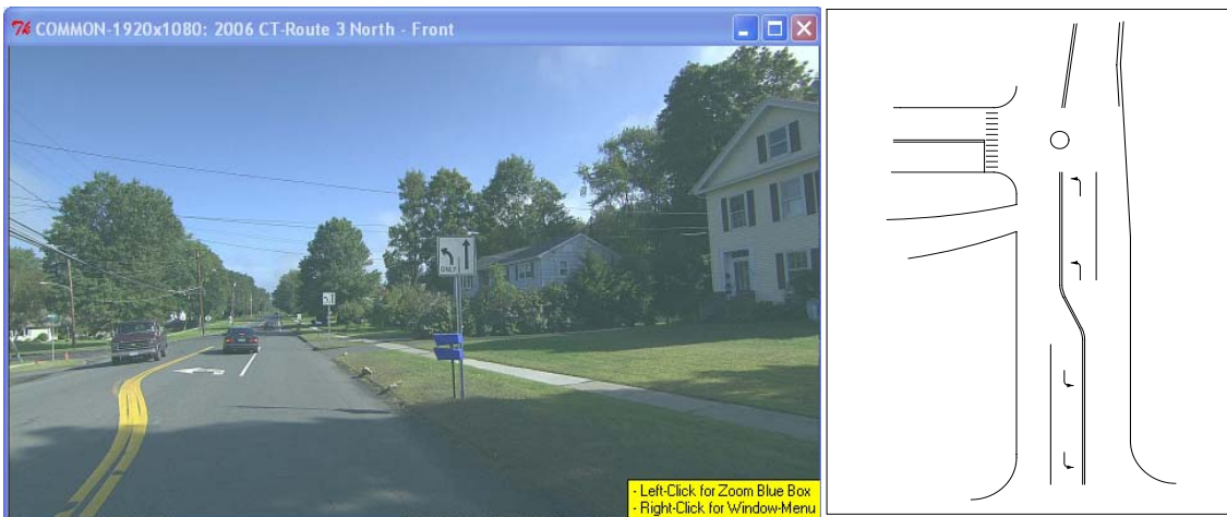
Example location with very short left turn lane taper and storage length
