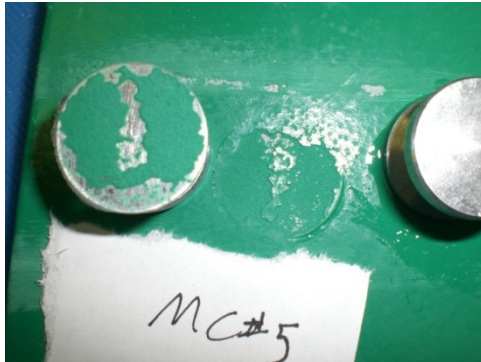
Figure 1. Paint B7-97 on metalized zinc after pull off at 700 psi.
