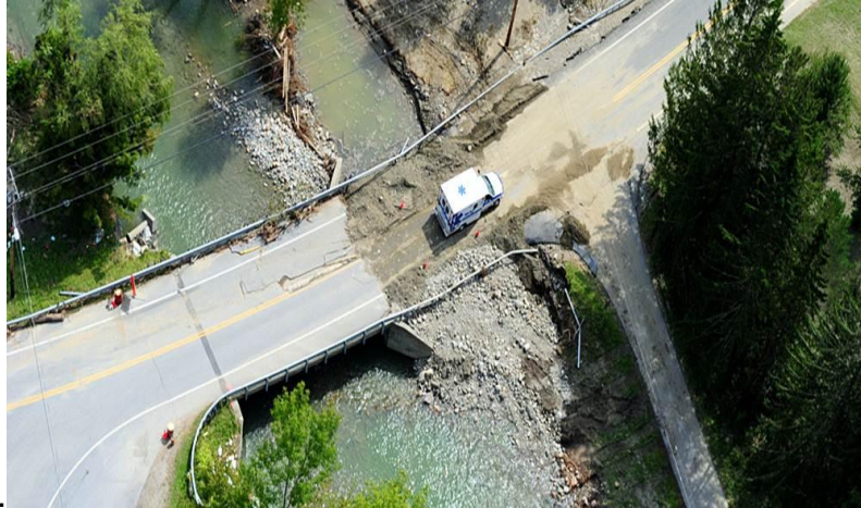
Figure 1. Bridge damage in southern Vermont as a result of flooding incurred during Hurricane Irene. Image source: Mansfield Flight LLC.
