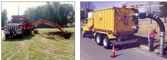
Culvert cleaning and drainage dredging, examples of costly BMP maintenance.
