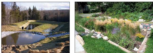
Two examples of stormwater best management practices: a wet pond on the left and a rain garden on the right ( http://www.maplewoodmn.gov/office.com ).
