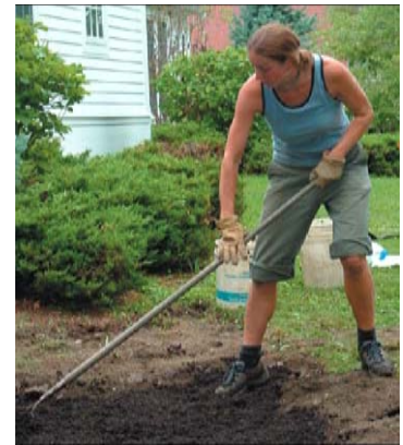
staff works on a rain garden at the Williston Town Library.
