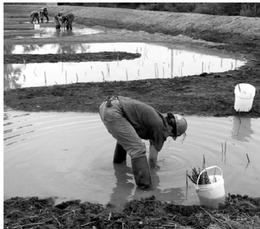
Vermont Youth Conservation Corps volunteers plant the Bartlett Brook stormwater treatment wetland.
