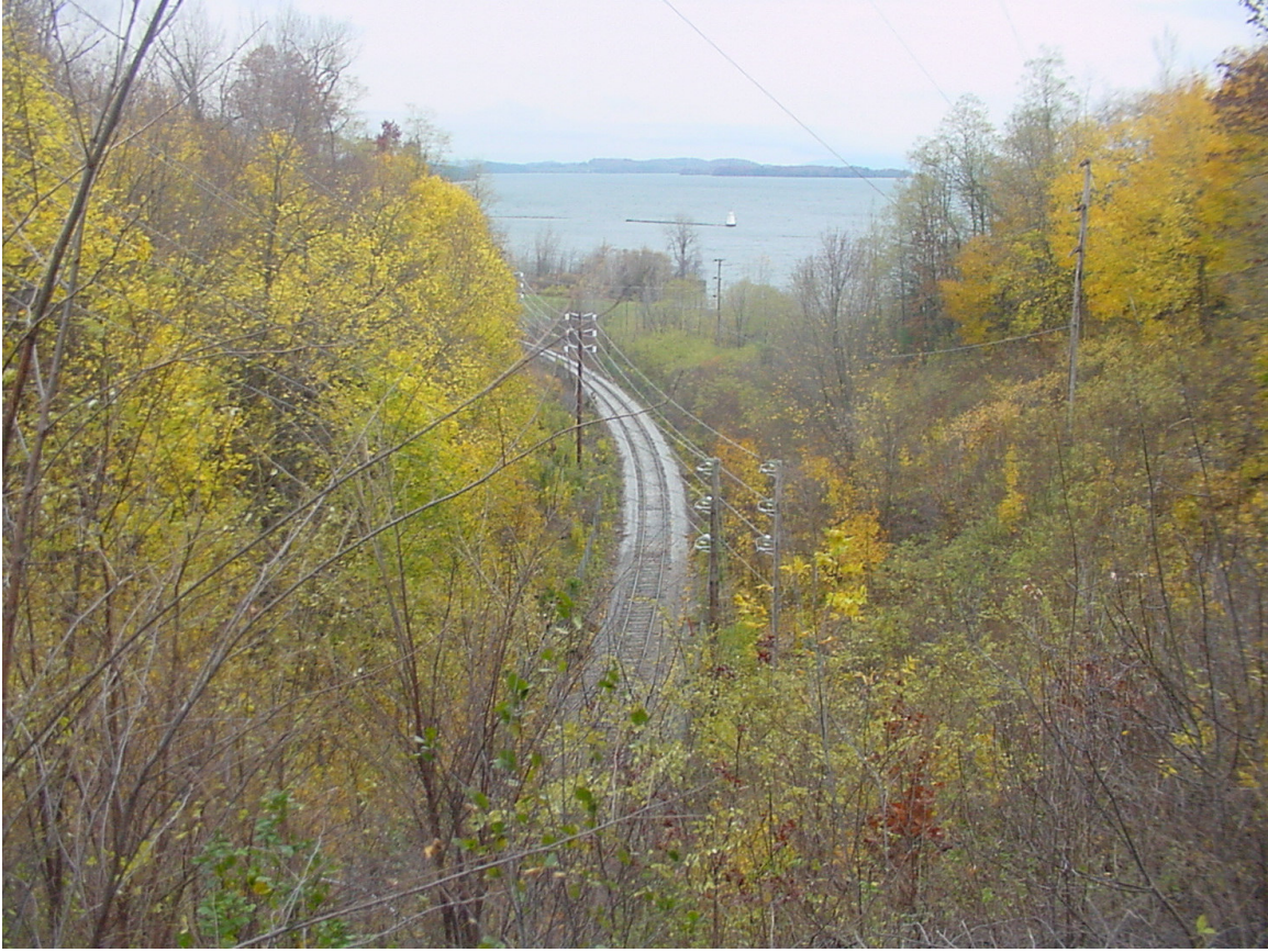
Figure 7b Shows the same view from above the tunnel shown in 7a as it stands today
