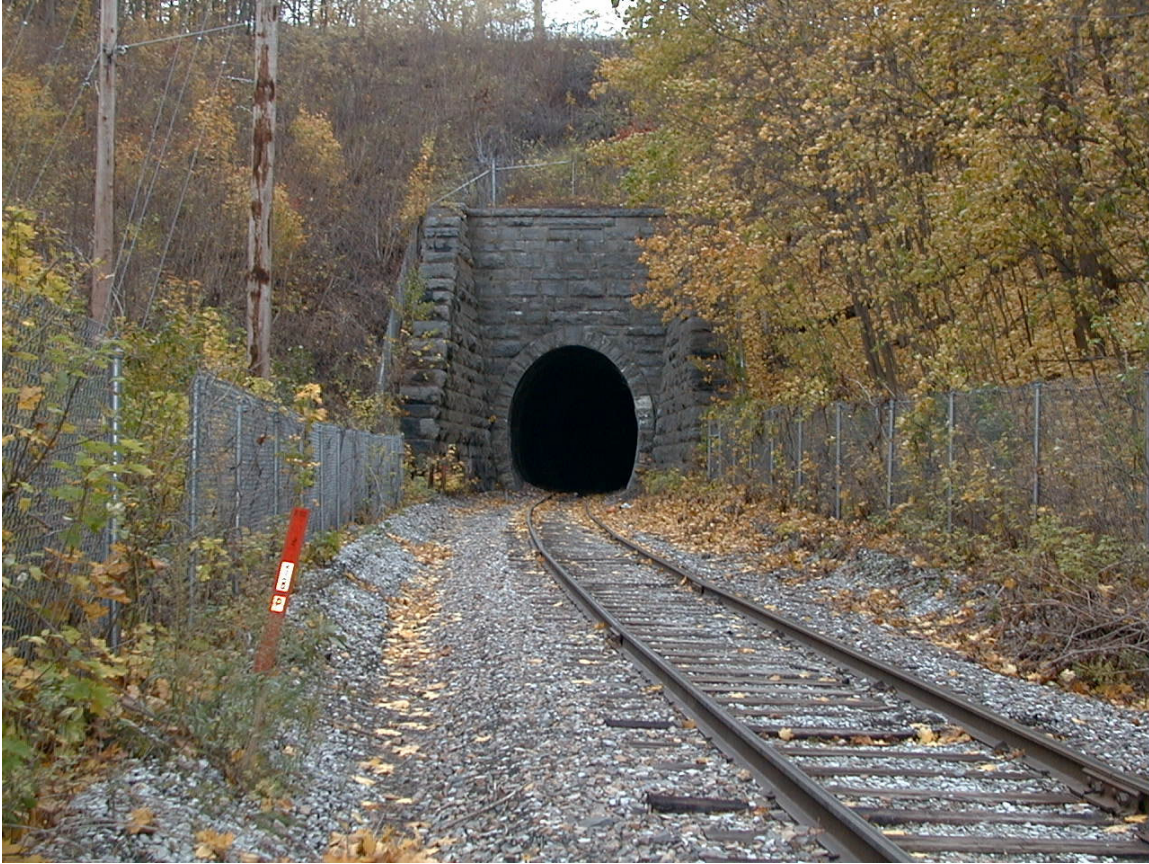
Figure 7c Shows the tunnel that stands today and is still used by trains.
