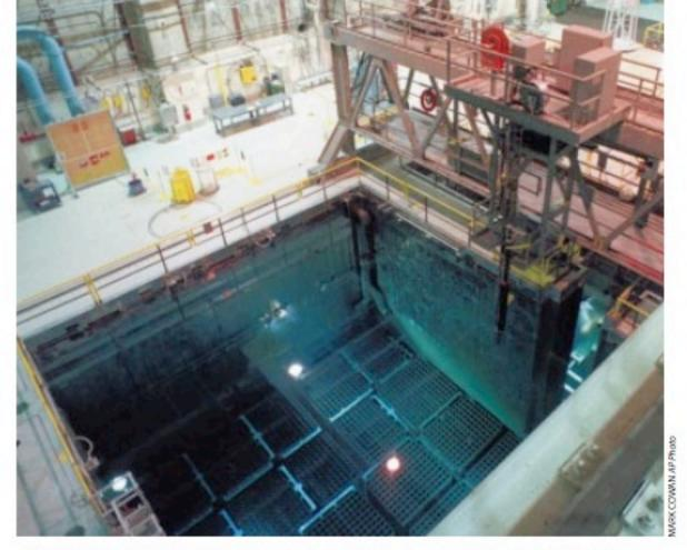
SPENT REACTOR FUEL will more than double in quantity in the U.S. by the year 2020, even if no new nuclear power plants are built, according to estimates of the Department of Energy (graph). Because no procedures for permanent disposal are yet established, the spent nuclear fuel is now stored temporarily at the reactor sites, often in cooling ponds (above).
