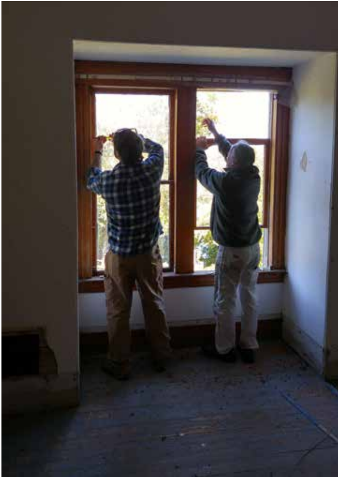
Participants at the window workshop removing and de-glazing windows at the Grand Isle Lake House
