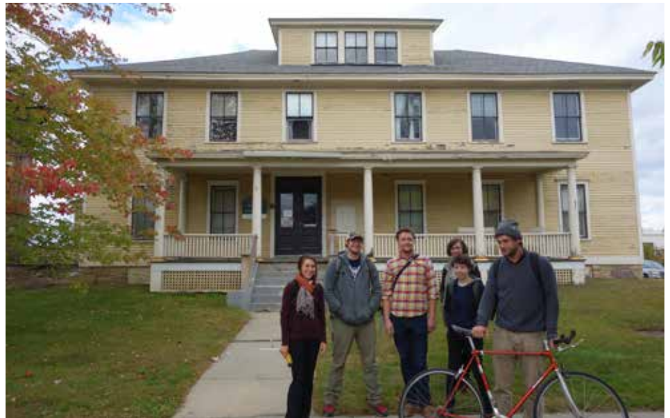
HP 206 class visiting 12 Colchester Avenue, one of the oldest buildings in Burlington
