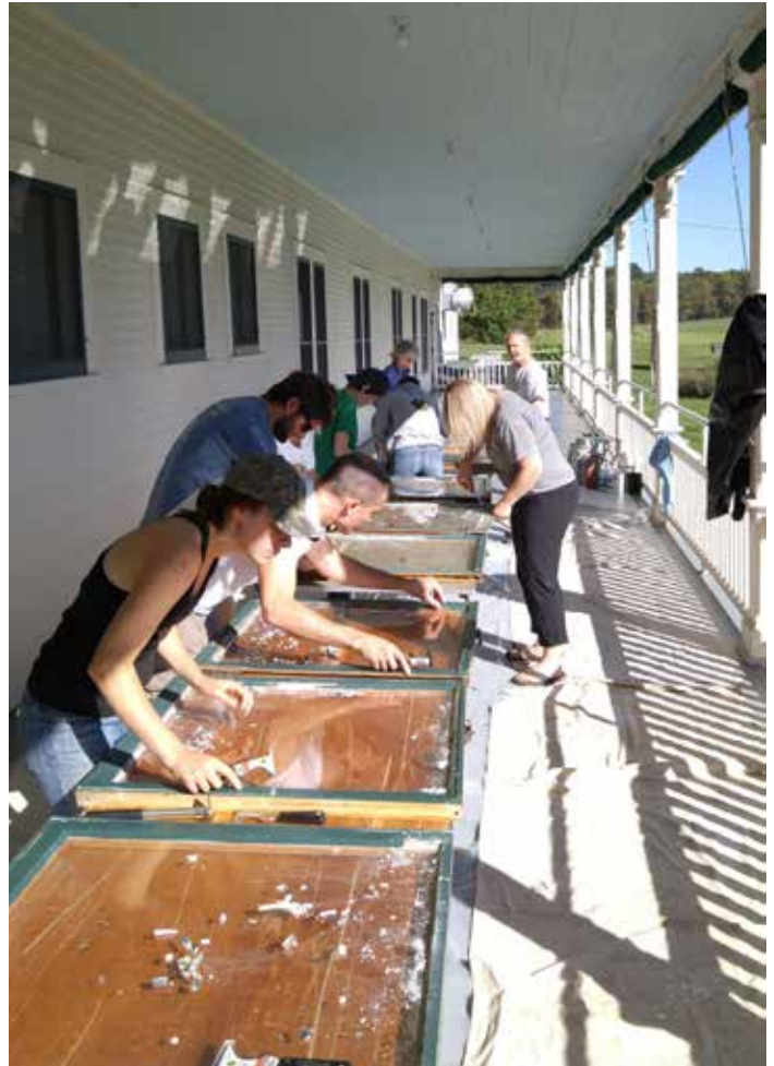
Participants at the window workshop removing and de-glazing windows at the Grand Isle Lake House
