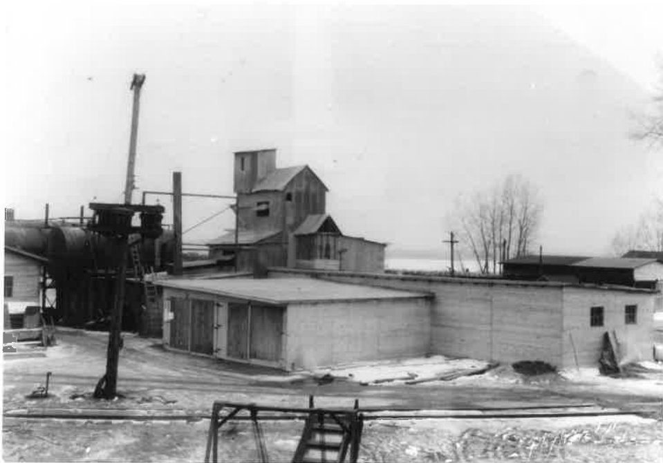
Fig. 24 This 1937 photo shows the Burlington Street Department's asphalt plant, looking west, after construction of sheds where concrete sewer pipe was cast. The original photo caption reads: "The long wing at the right has a platform through the center from which the concrete is poured from two-wheeled buggies into the steel form placed on both sides. The wing at left is the curing room where the tiles were stored for a period of 48 hours before being taken onto the job. Both buildings were equipped with steam heat." (Source: MacAllister Photo Collection, Wilbur Special Collections, Bailey-Howe Library, Burlington, Vermont, 1932.)
