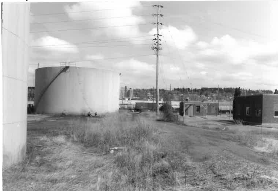
Fig. 7 This photo shows the sludge storage tanks located in the old boat slip looking east toward Battery Street. The building visible on the right is the control building. (Photo: Thomas Visser, April, 1990)
