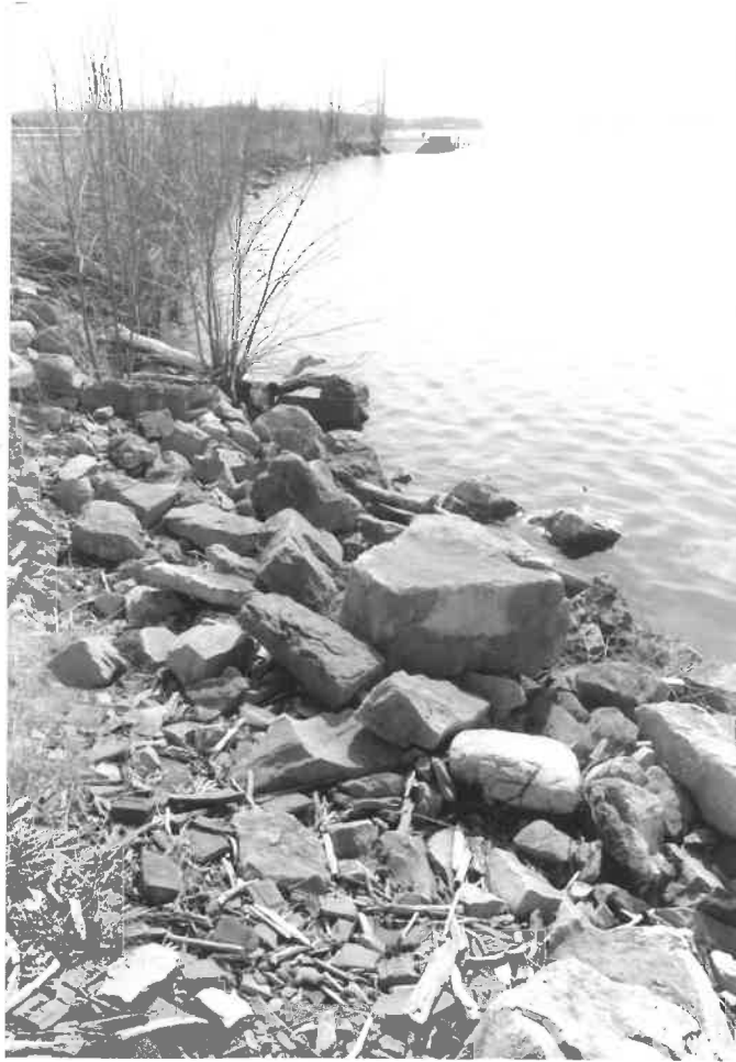
Fig. 3 This photo shows the shoreline of the wastewater treatment plant site looking south from near the northern terminus of the property. In the foreground, driftwood and other debris are visible intermingled with the crushed stone of the lake barrier. (Photo: Thomas Visser, April, 1990)
