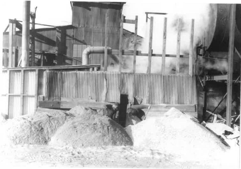
Fig. 20 This 1937 photo shows the types of possible evidence that may be found on the site remaining from the operation of the asphalt plant. The mounds on the left appear to be sand, and the pile on the right appears to be crushed stone. (Source: MacAllister Photo Collection, Wilbur Special Collections, Bailey-Howe Library, Burlington, Vermont, 1937.)
