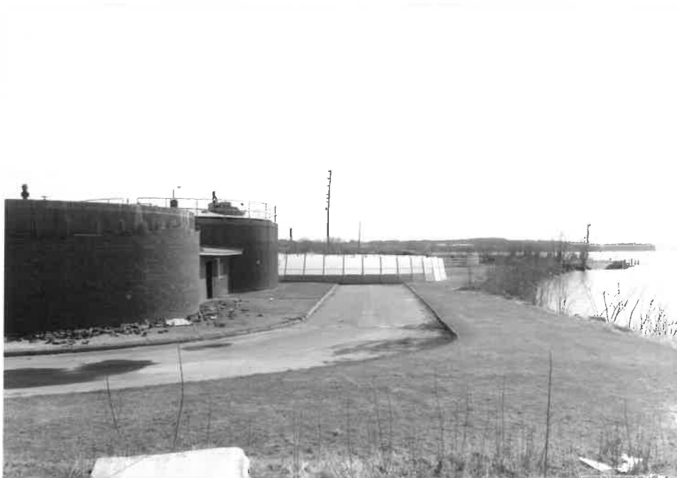
Fig. 5 This photo is looking south from the old boat slip. On the left are the digesters and behind them the aeration tanks. In the distance the sewer outfalls are visible. (Photo: Thomas Visser, April, 1990).
