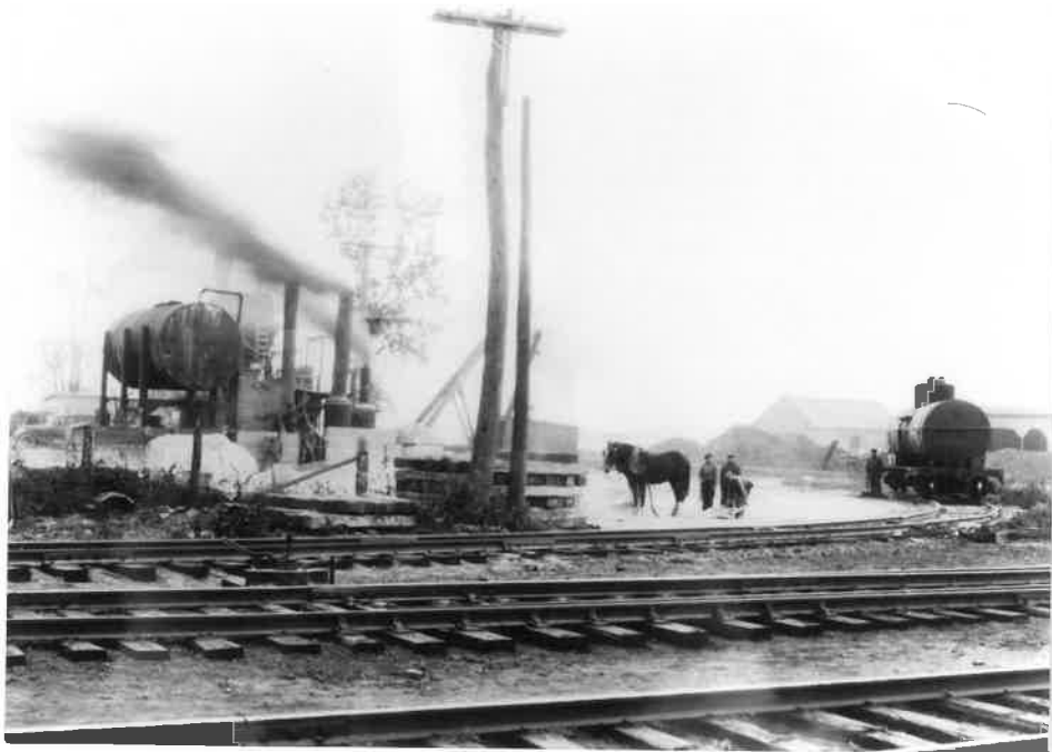
Fig. 18 This 1929 photo, looking west, taken after the construction of the asphalt plant, shows the rail spur and, behind the horse, the boat slip. The rail spur ran along the edge of the slip to the dog leg derricks behind the pole, which transferred stone and other goods between the boats at the dock and the waiting train cars. (Source: McAllister Photo Collection, Wilbur Special Collections, Bailey-Howe Library, Burlington, Vermont, 1929.)
