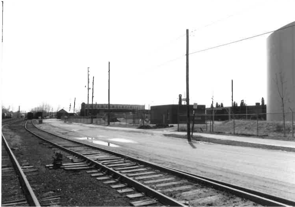
Fig. 1 This photo looking south shows the track of the Vermont Railway running along the eastern boundary of the sewage treatment plant site. The road immediately west of the tracks may follow the original, pre-fill shoreline. (Photo: Thomas Visser, 1990)
