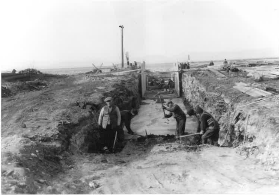
Fig. 19 In this 1932 photo, the sidewalls of the trench for the main trunkline sewer reveal the layering of fill deposits. This is especially noticeable along the left wall next to the man looking at the camera. (Source: MacAllister Photo Collection, Wilbur Special Collections, Bailey-Howe Library, Burlington, Vermont, 1932.)
