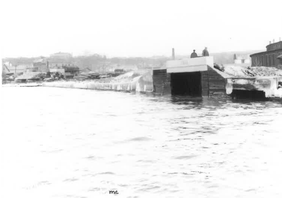
Fig. 6 This 1932 photo shows the newly constructed sewer outfall with its dated, concrete header next to the old 1894/1914 sewer outfall. The asphalt plant is visible on the far left, and the roundhouse of the Rutland Railroad is on the far right. (Source: MacAllister Photo Collection, Wilbur Special Collections, Bailey-Howe Library, Burlington, Vermont, 1932.)
