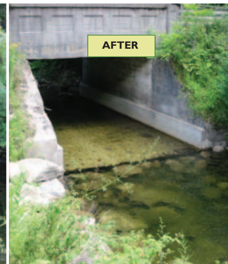
The Friends of the Winooski retrofitted this stream crossing to eliminate the dropoff from the culvert, reduce stream velocity, and increase depth, improving passage for fish and other aquatic organisms.
