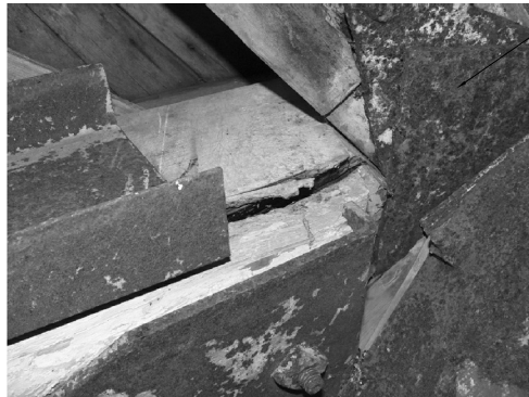
VALLEY RAFTER 17 NORTH, ABOVE DRILLING LOCATION D12 WITH A SPLIT END
