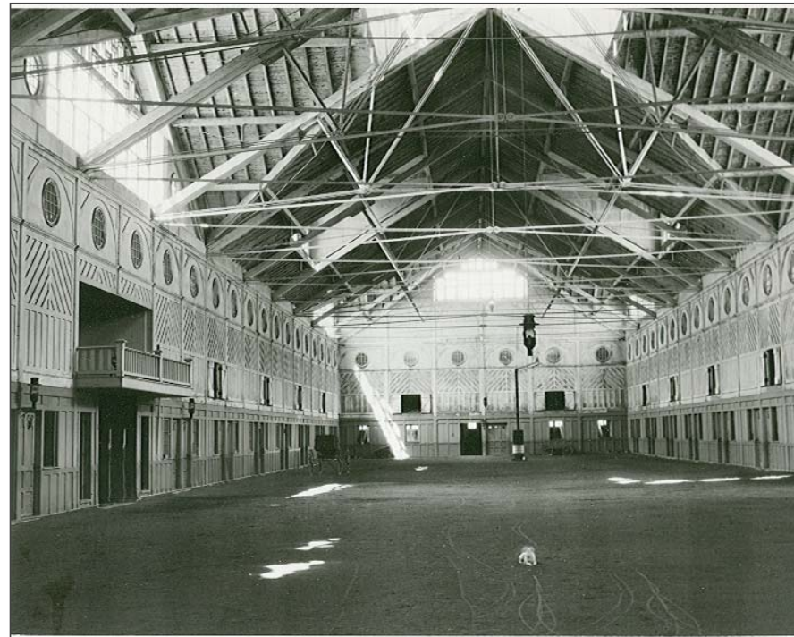
Figure 2: The Breeding Barn interior exhibits an extraordinary level of interior finish. The use of iron rather than wood for truss elements except top chords helps to convey the impression of great volume in the riding ring space.
