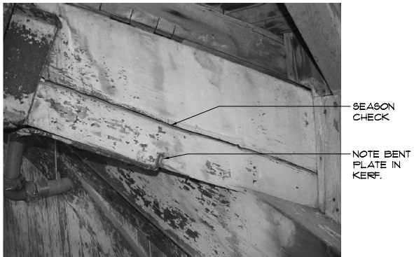
4 VALLEY RAFTER 1 SOUTH, SEASON CHECK IN THE SOUTH FACE PI.1 NOT TO SCALE
