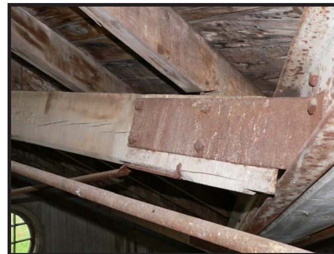
Figure 30. Upper purlin twisted at junction with Valley Rafter 11 South.
