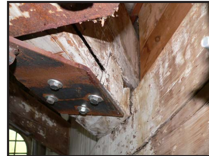
Figure 10. Valley Rafter 1 North at east wall; note deformed lags.
