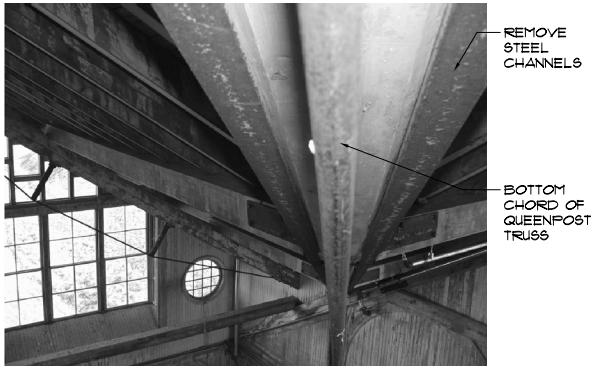
1 VALLEY RAFTER 1 NORTH VIEWED FROM THE APEX PI.1 NOT TO SCALE
