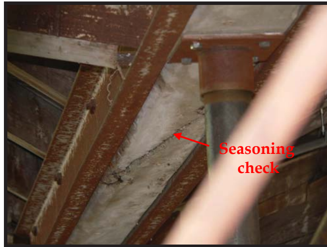
Figure 20. Seasoning check indicating severe slope of grain (1.5" in 10") in Valley Rafter 4.5 South.
