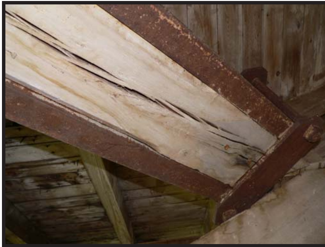
Figure 27. Valley Rafter 11 North showing seasoning checks.
