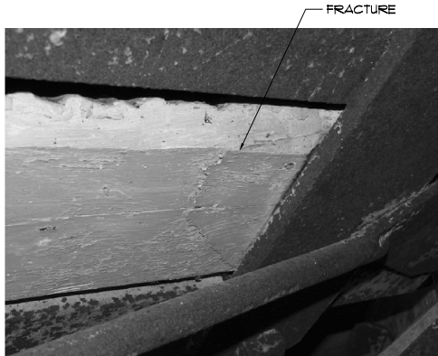
FRACTURE NEAR THE APEX OF VALLEY RAFTER 17 NORTH BELOW THE END SPLIT SHOWN IN 3/P1.3
