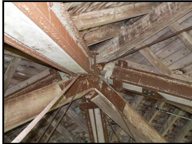
Figure 6. Apex of valley rafters showing steel side channels, east end of the Barn.
