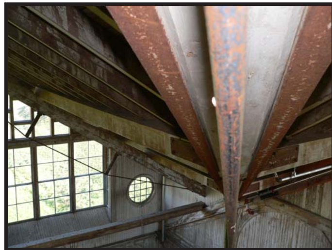
Figure 9. Valley Rafter 1 North viewed from the apex.
