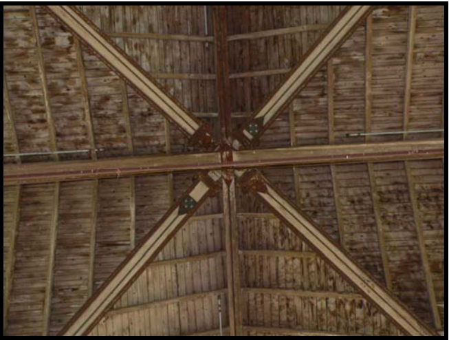
Figure 5. Apex of valley rafters, east end of the Barn.
