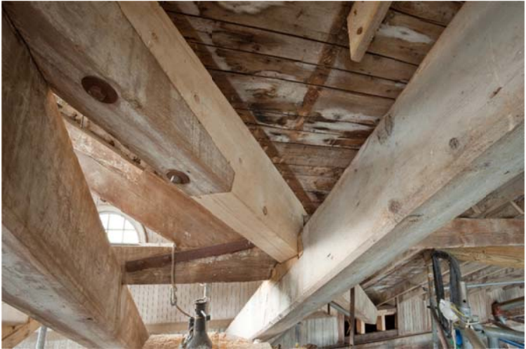
Figure 13 – New timber was scarfed into the valley member at J14.5 where both timbers receive support from truss rafters. The length of the replacement timber is approximately 6.4 m.
