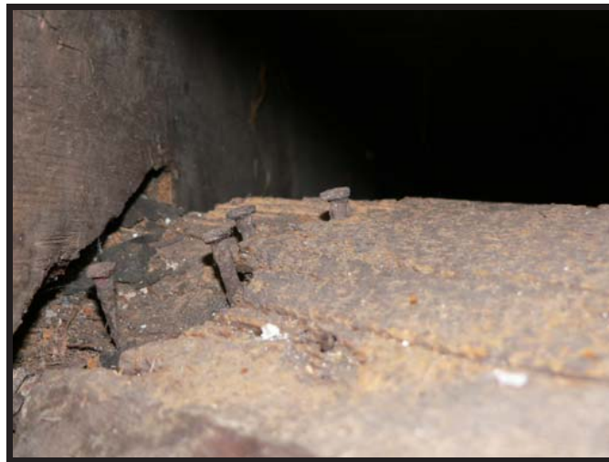
Figure 17. Heel of Valley Rafter 4.5 North; note corroded nails not fully securing the rafter to the top plate.
