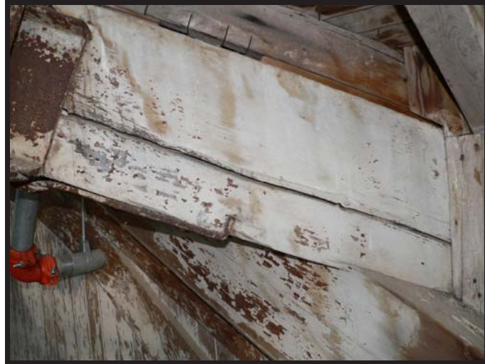
Figure 13. Valley rafter 1 South, drying check on the south face.
