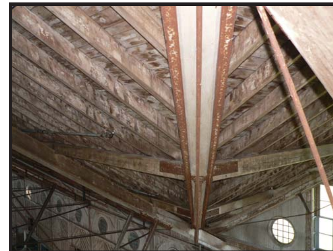
Figure 15. Valley Rafter 4.5 North viewed from the apex.
