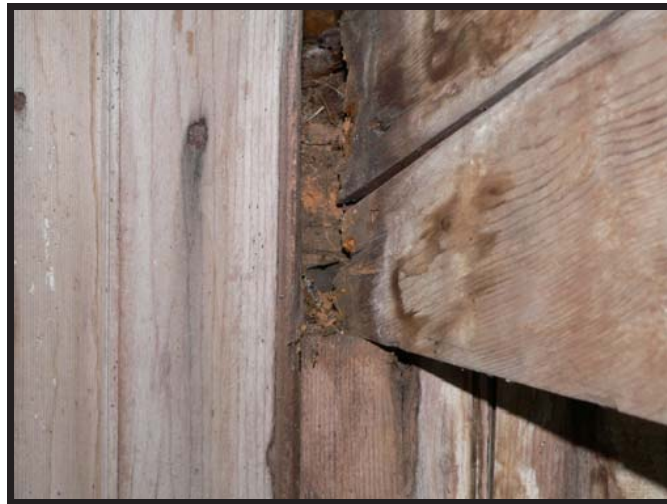
Figure 16. Heel of Valley Rafter 4.5 North at the north wall showing decay in rafter and top plate.
