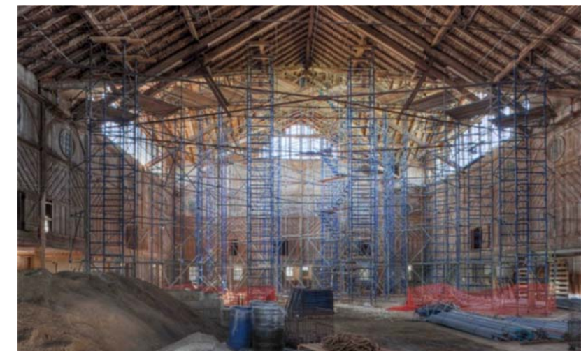
Figure 11 – Scaffolding used for accessing the roof was X-shaped in plan (top) and surrounded by structural staging that supported purlin loads (bottom).
