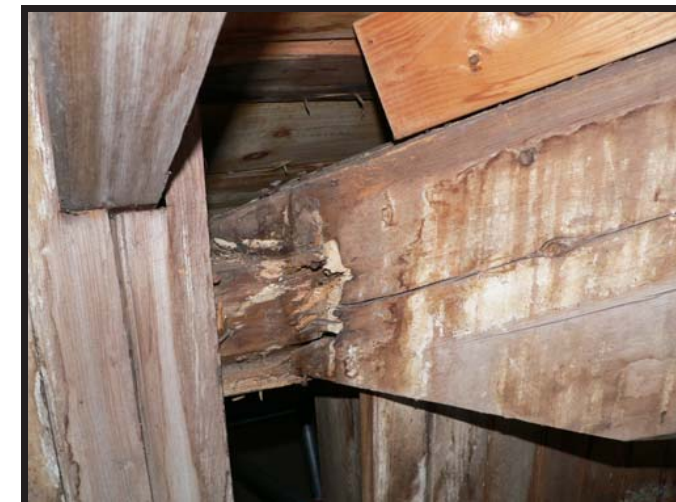
Figure 34. Valley Rafter 14.5 North showing decay in the rafter and the top plate of the interior wall.
