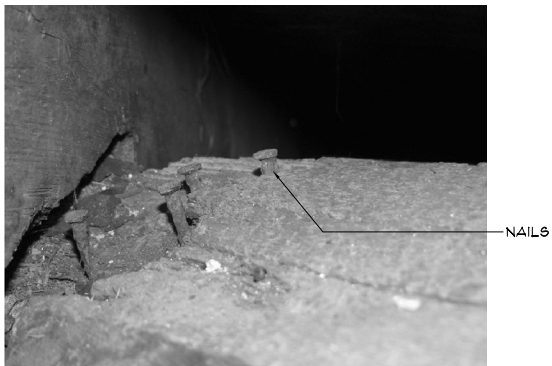
7 HEEL OF VALLEY RAFTER 4.5 NORTH, NOTE CORRODED NAILS NOT FULLY SECURING THE RAFTER TO THE TOP PLATE PI.1 NOT TO SCALE
