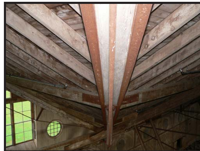
Figure 32. Valley Rafter 14.5 North from peak viewed from the apex.
