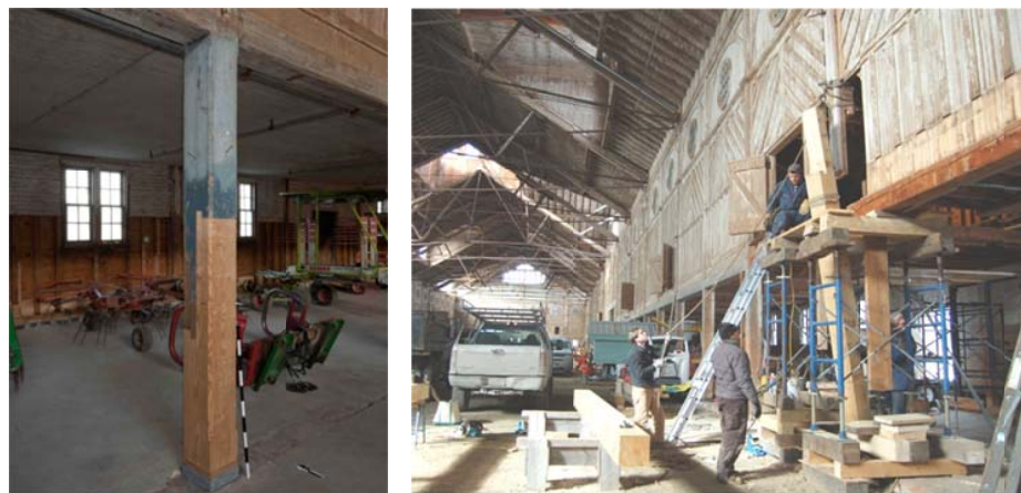
Figure 10 – Columns were repaired by scarfing in new timber to replace decayed portions, using a nosed scarf form found elsewhere in the barn. New column bases were placed on limestone plinths and white oak shims, elevating them above a mid-20 th century concrete floor (left). In four cases, column splices were made at the aisle level, requiring renewal of girt joinery and, in this case, replacement of the girts on either side (right).
