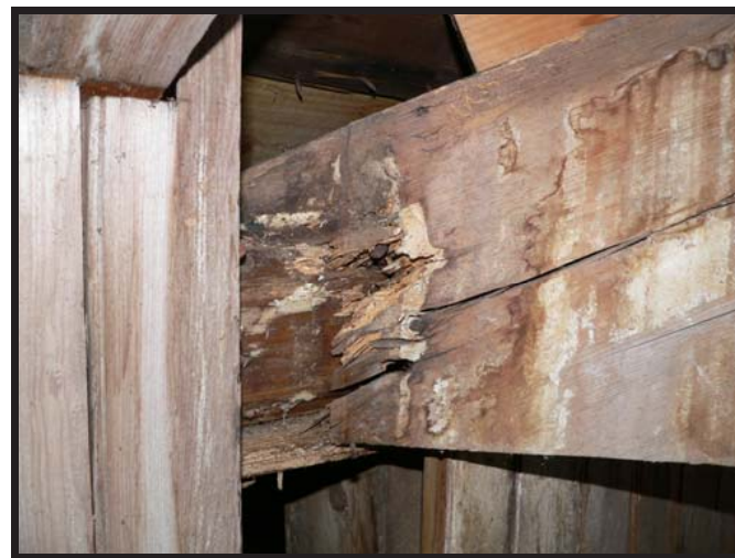
Figure 39. Valley Rafter 14.5 South at the top plate of the interior wall.
