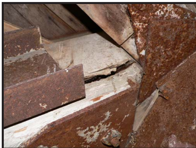
Figure 44. Valley Rafter 17 North, above drilling location D12 showing end split.
