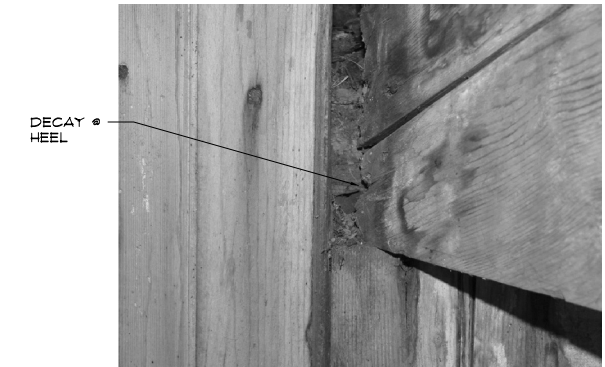
6 HEEL OF VALLEY RAFTER 4.5 NORTH AT THE NORTH WALL SHOWING DECAY IN THE RAFTER AND TOP PLATE PI.1 NOT TO SCALE
