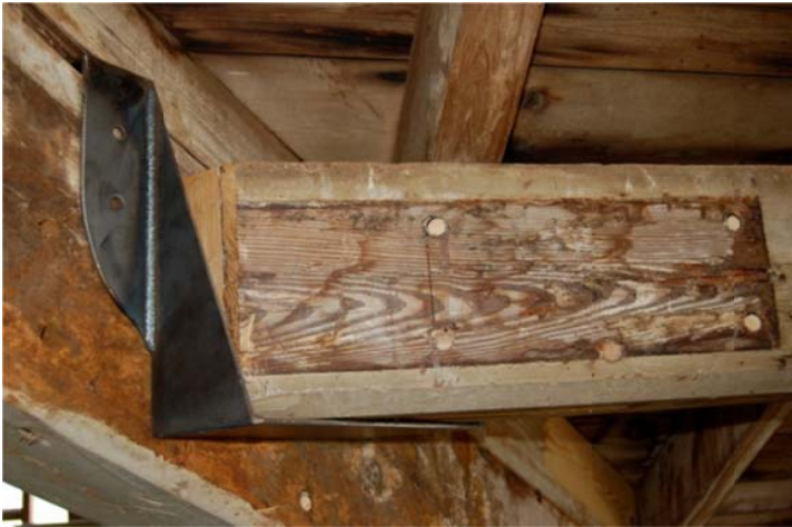
Figure 17 – Purlins are supported on custom-made bridles that replicate original ironwork. Where it was necessary to extend purlins, loose tenons were installed and blocks added to brace the valley timber.
