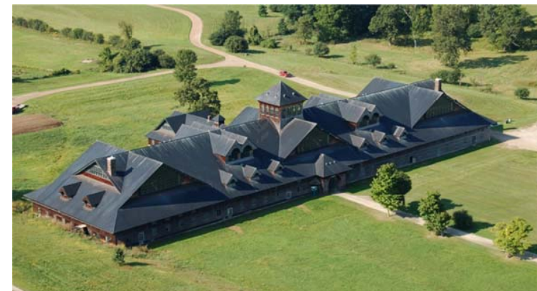
Figure 1 – The Breeding Barn at Shelburne Farms, a National Historic Landmark, is dominated by its complex-sloped 8094 m 2 hipped roof with multiple dormers and an enormous central lantern.
