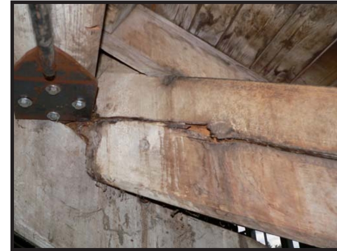
Figure 33. Failure in Valley Rafter 14.5 North, east of supplemental truss.
