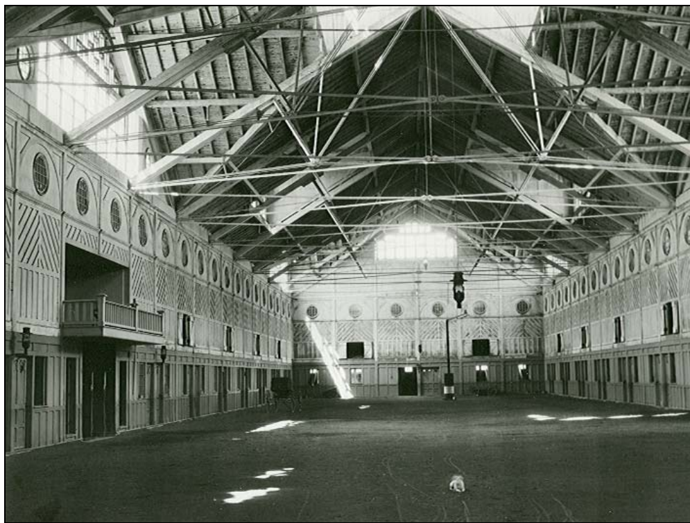
Figure 4. Barn interior.c1900 showing the roof frame of the riding ring, including iron cross-brace ties. Shelburne Farms Archives. All rights reserved. May not be reproduced without permission.
