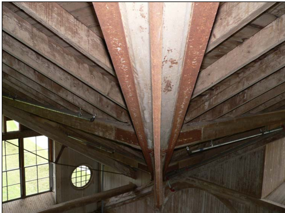
Figure 5. Valley Rafter 17 South viewed from the apex.
