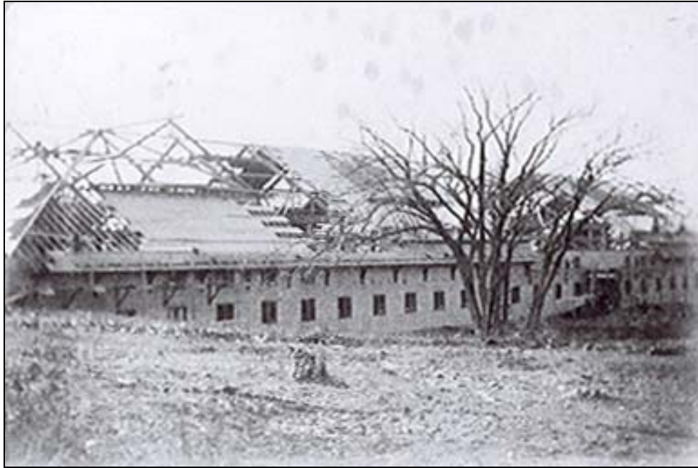
Figure 2. The barn under construction, c1890.
