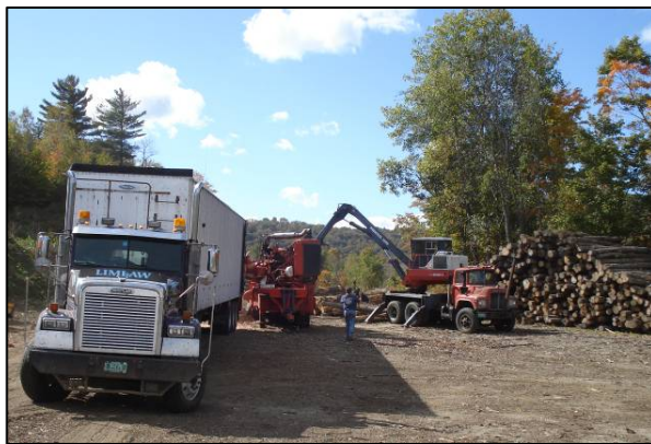
Low-grade roundwood is trucked from harvest sites to Limlaw's storage yard where it is periodically chipped into trailers for final delivery
