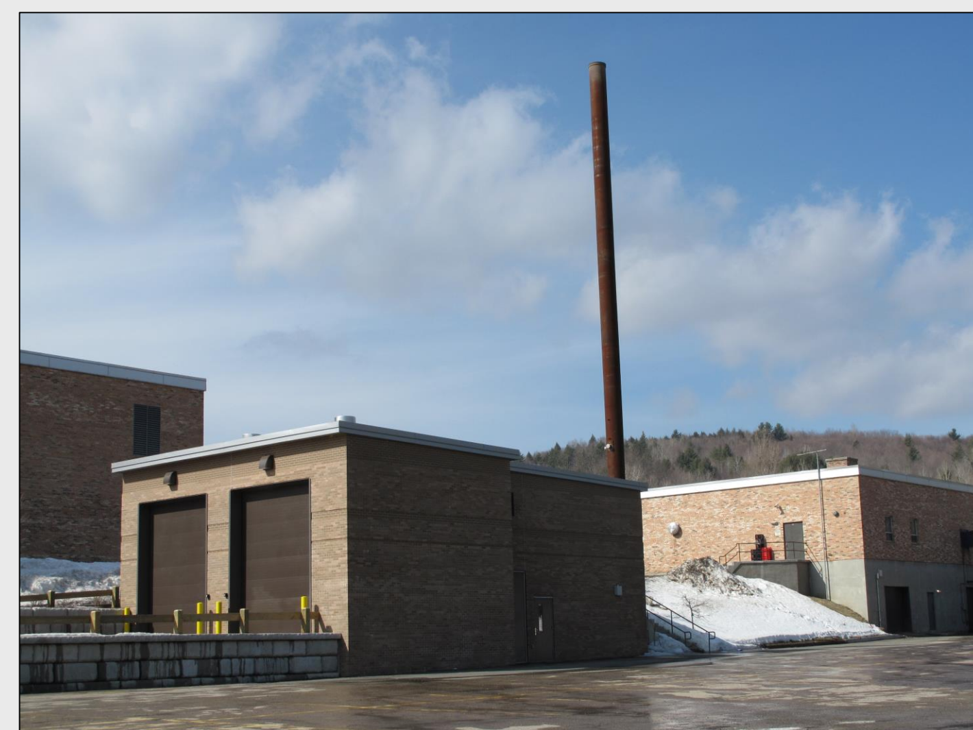
Harwood Union High School's wood-chip-based heating facility, Moretown, Vermont
