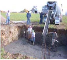
From the beginning, this system encountered problems. After building a reinforced 4' deep by 21' square concrete base for his new 10,000 pound wind tower, he discovered that the tower's feet did not align properly with the footings he had been instructed to build. He hired a welder to fix the problem.
