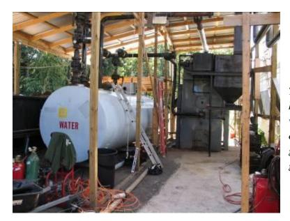
The 3 million Btu Conifer furnace heats water in the Kewanee boiler; valves are set to control how much of the hot water is sent to heat the greenhouse or stored in the 3,000 gallon reservoir.
