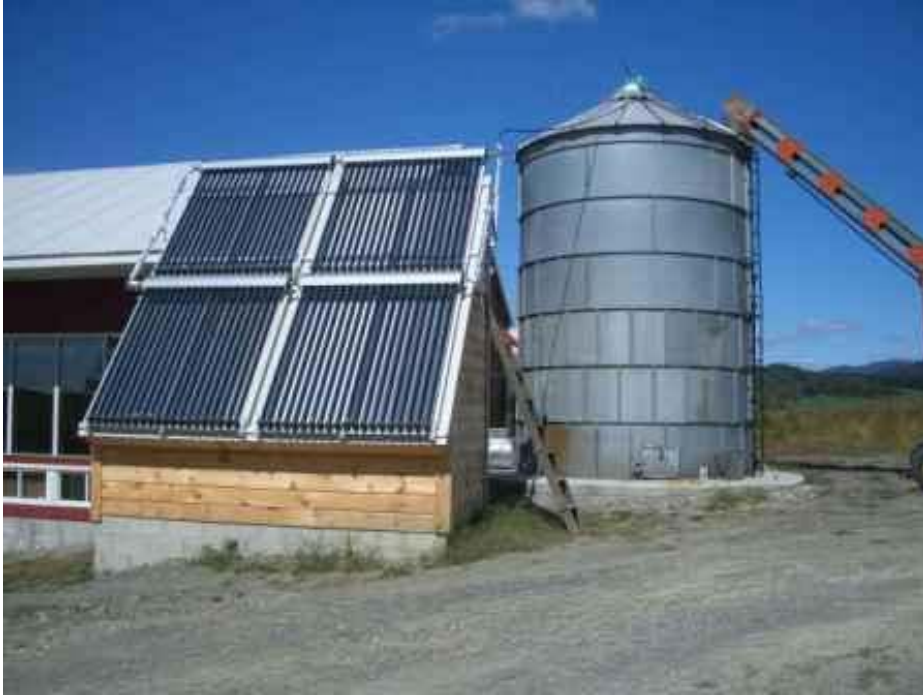
Figure 8 - Example of evacuated tube solar collector installed at State Line Farm in Shaftsbury, VT. This was a 4 panel (80 tube) system purchased from SunMaxx Solar in Bainbridge, NY.
