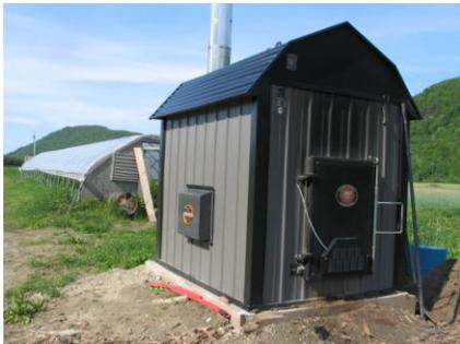
The outdoor wood boiler at Blais Farm is from Central Boiler, Greenbush, MN ([www.centralboiler.com](http://www.centralboiler.com)). It is one of largest models they make, the Classic CL7260, with a 764-gallon water reservoir and a firebox that measures 72x60x40 inches. It is located well away from the house and road, at the edge of a field by the greenhouses. Insulated underground pipe carries hot water from the furnace to the various structures and into heat exchangers that release the heat.
