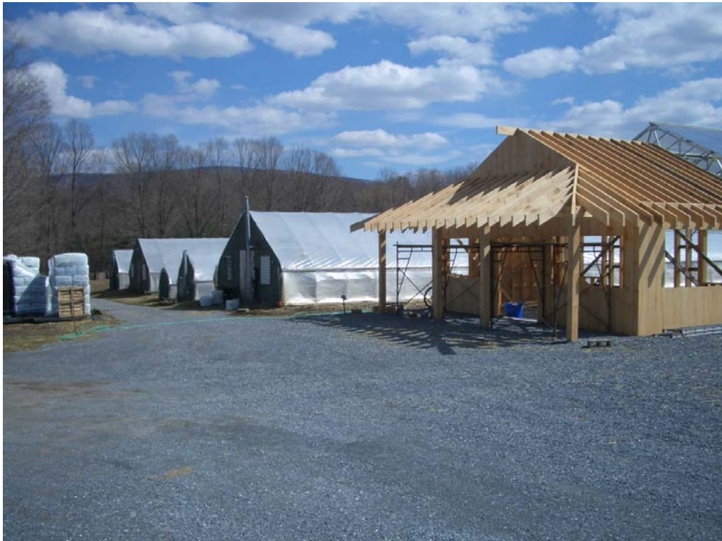
Figure 1 A view looking southeast showing the display house under construction and also houses #1-5. The display house was completed in the Fall of 2009.
