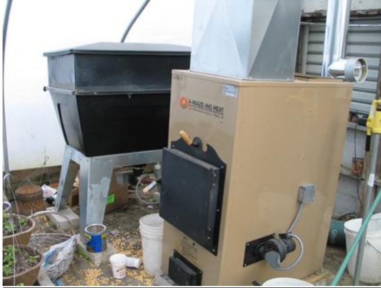
Figure 11 - The LDJ Amaize-ing Furnace at Harlow Farm with a hopper extended to hold 21 bushels vs 14 in the default version.
