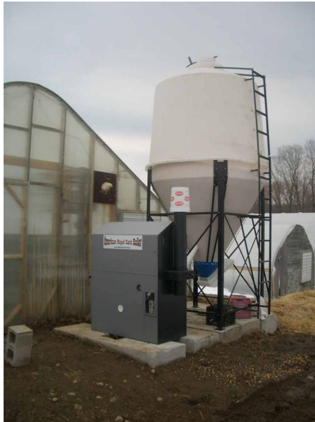
Figure 16 - The American Royal multifuel boiler and hopper at Clearbrook Farm.
