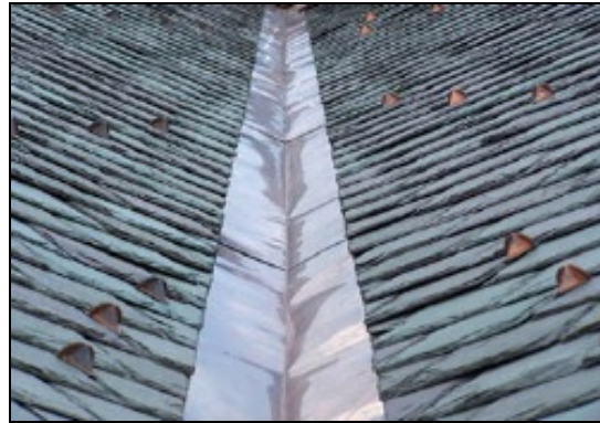
Linear progress: Exterior work on the new Dudley H. Davis Center, including the installation of these Vermont-produced slate roof tiles, is anticipated to be largely complete at the end of December. (Image: Courtesy of the Davis Center)
