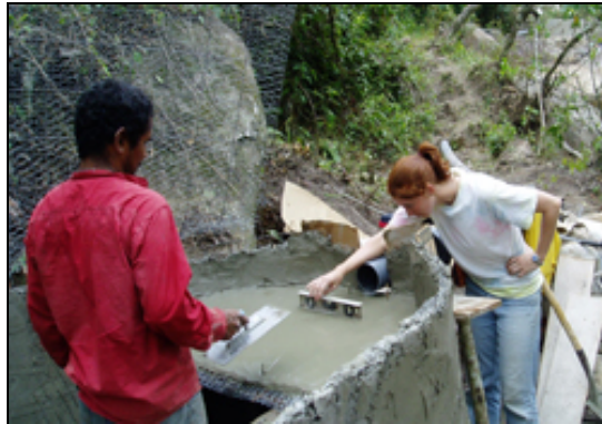
Nicole Mason '07 designed and installed a sediment catch basin in Honduras that has greatly improved the water quality of a small town. (Photo: Courtesy: Dan Baker)
