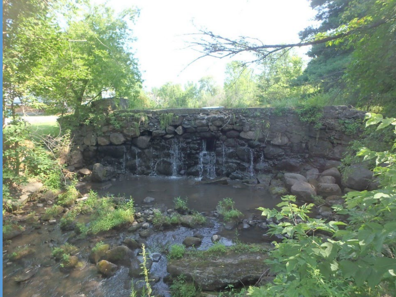
Looking Upstream at Old Stone Dam 2017
