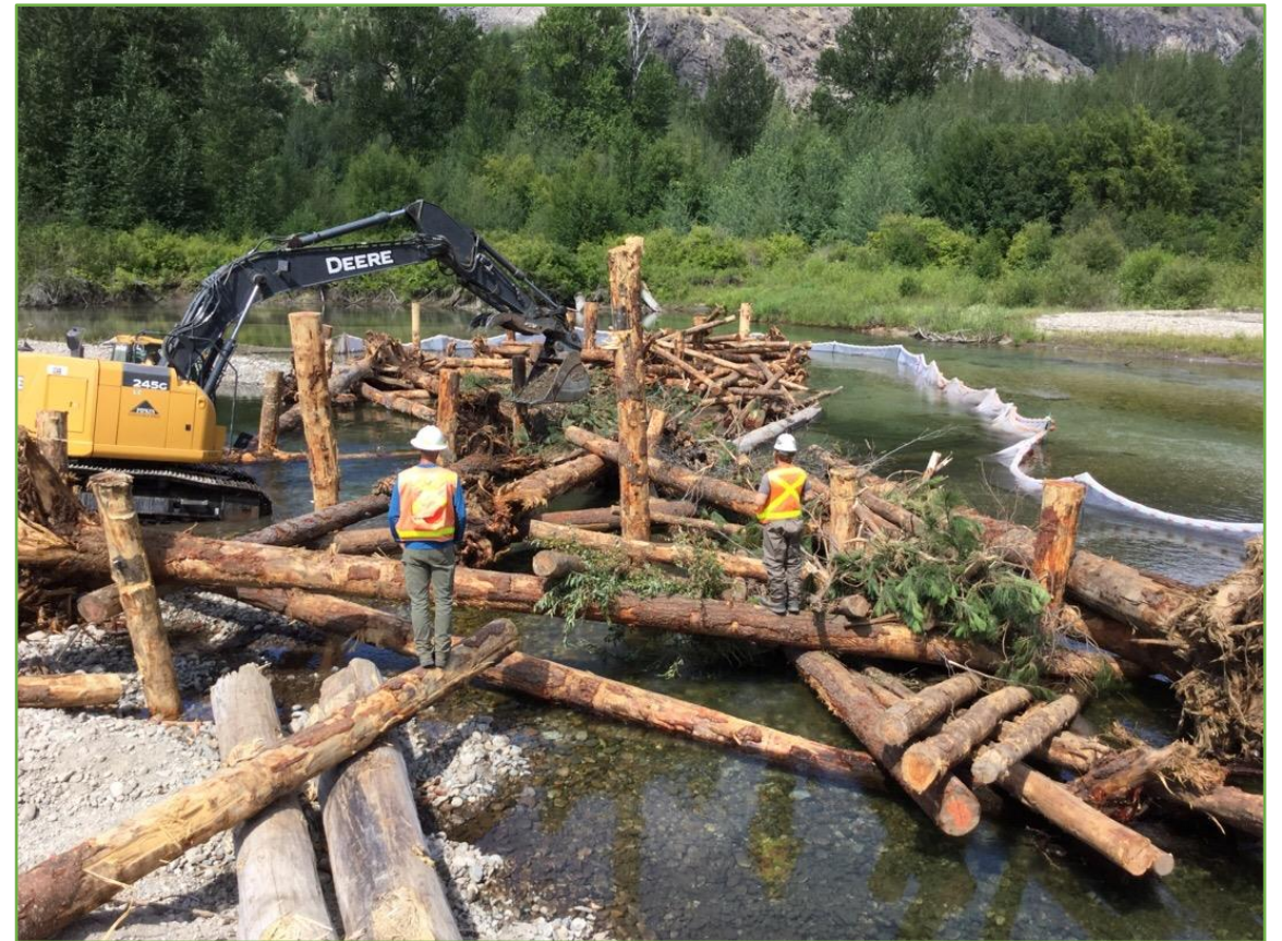
Engineered Log Jams (ELJ), Entiat River, WA
