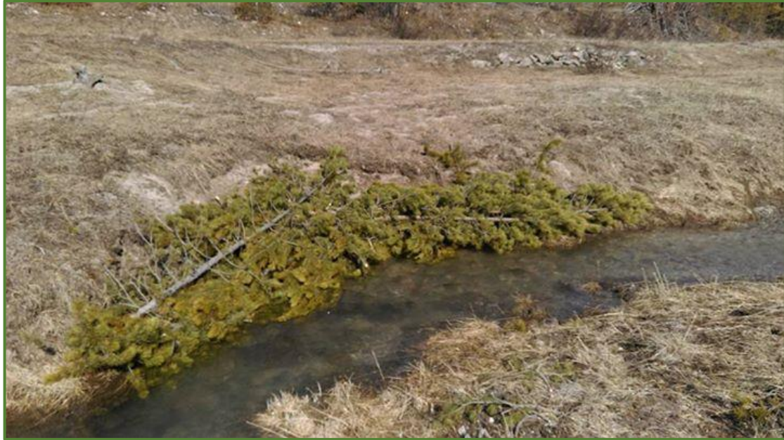
Brush fascines for bank stabilization, Mill Creek, MT
