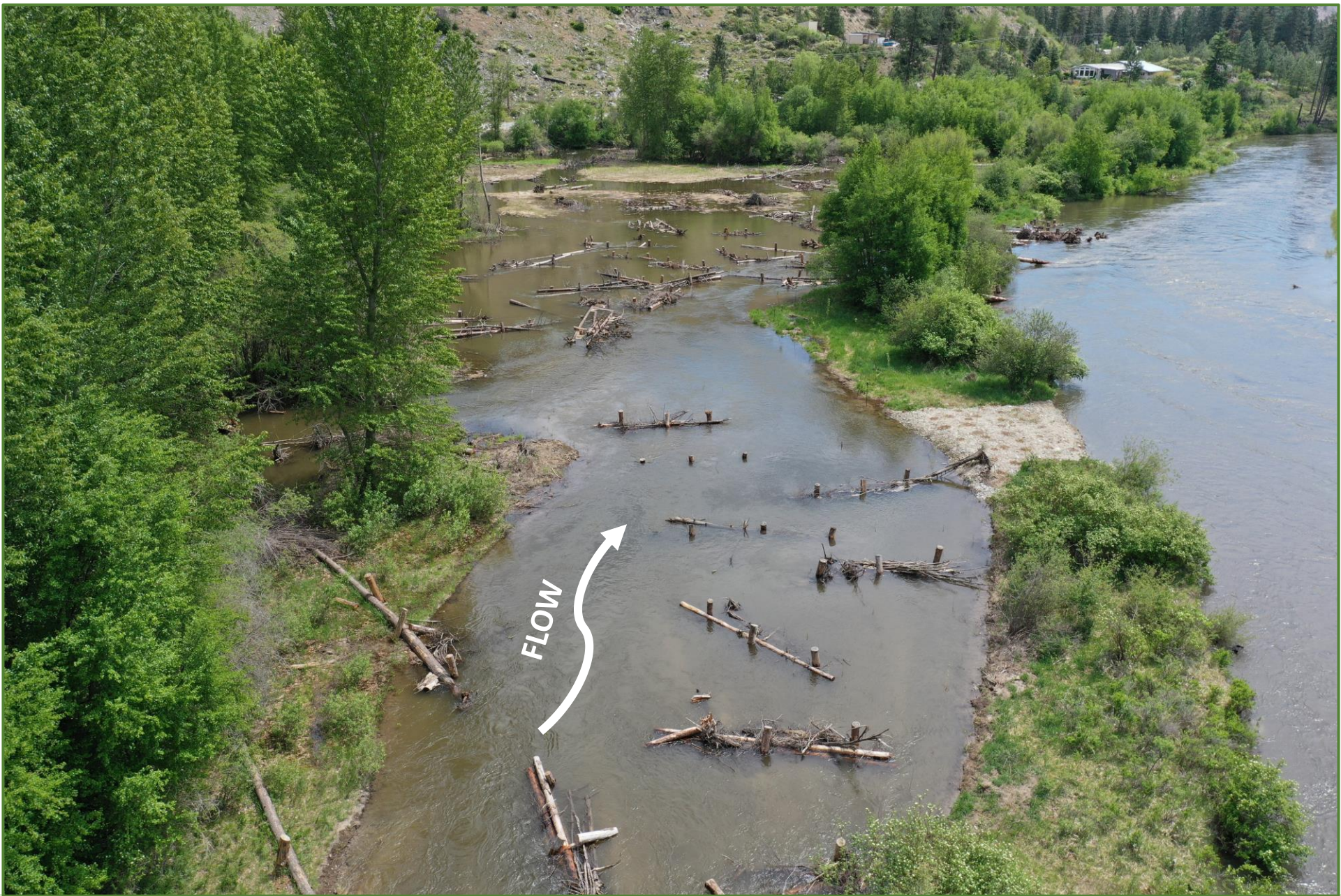
Post-Assisted Log Structures (PALS), Entiat River, WA
