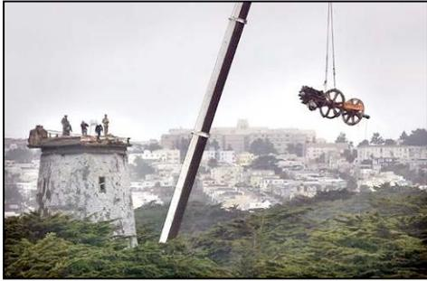
**Figure 21. Removal of antique gear mechanism via crane, June 26, 2002 (Scott Sommerdorf, San Francisco Chronicle)**
