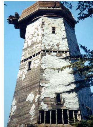
**Figure 18. Murphy Windmill in 2002 showing exposed wood cladding and shingle loss**
