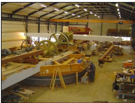
**Figure 22. Restoration of cap in the Netherlands (Campaign to Save the Golden Gate Park Windmills)**
