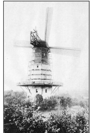
**Figure 8. Windmill under construction (California Historical Society FN-32851)**
