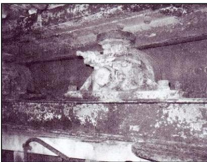
**Figure 19. Severely deteriorated iron and steel mechanism inside the Murphy Windmill (Carey & Co.)**
