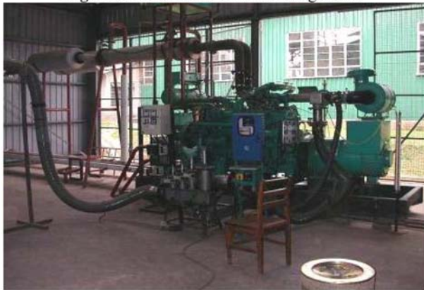
Figure 4: 250 kW producer-gas engine with heat exchangers (upper left corner at exhaust pipe, heat exchanger at cooling cycle covered by control units).
