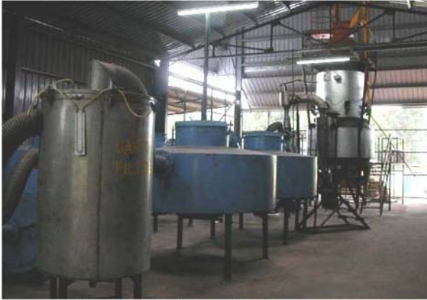
Figure 3: Filter line and WBG 400 gasifier.
