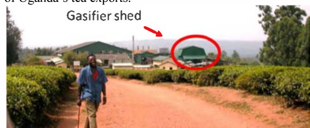
Figure 1: Muzizi Tea Estate processing facility with gasifier shed.
