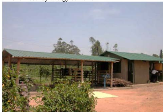
Figure 7: Gasifier shed with fuelwood storage and processing shed attached.
